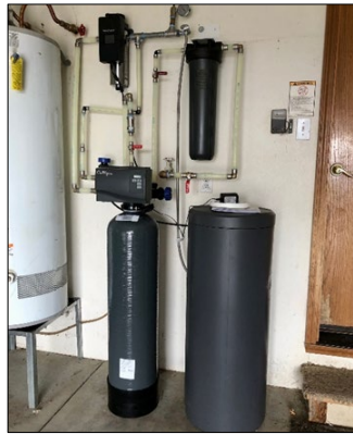
(Above) An Army contractor connects a UV system to the first POET filtration system installed in an East Selah, home where PFAS levels are at or above 70 ppt.
