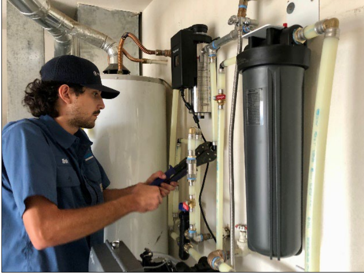
(Above) An Army contractor connects a UV system to the first POET filtration system installed in an East Selah, home where PFAS levels are at or above 70 ppt.
