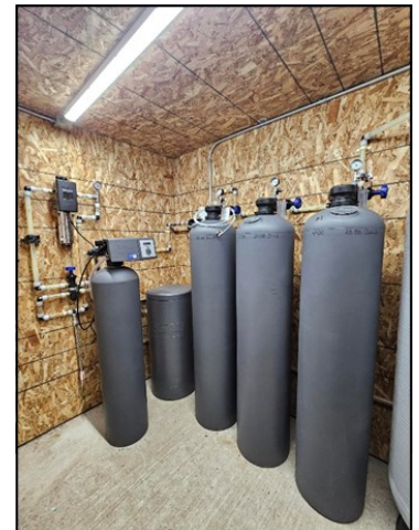
Some components in a single-family POET system.
