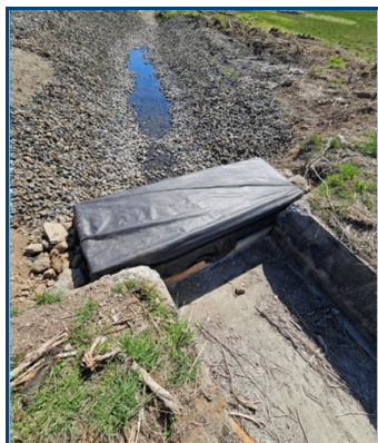
Overshoot of Roza Canal with RCM barrier in place.
