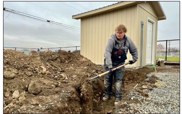
A contractor covers electrical conduit running power to a POET shed.
