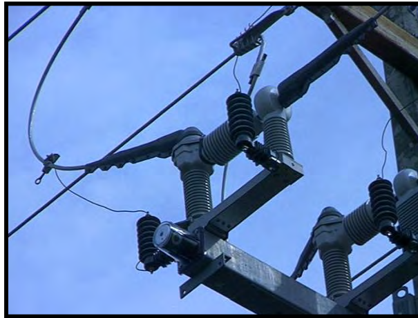
Figure 8-90. Switch with built-in animal protection.
