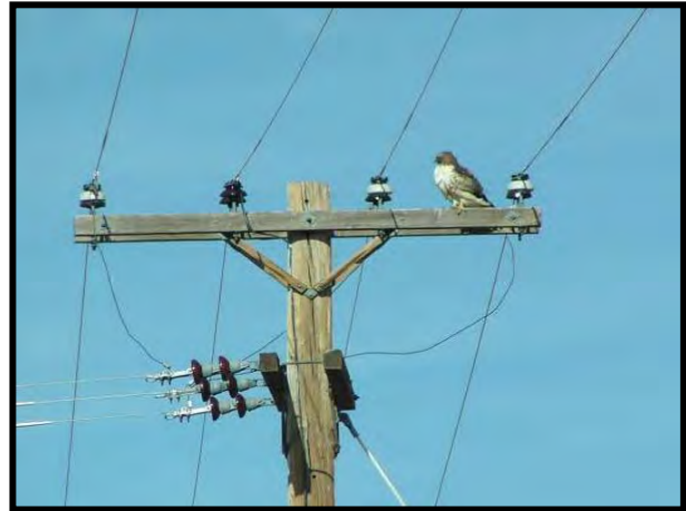
Figure 8-5. Flat-top unit provides inadequate separation (40 inches) for hawks.
