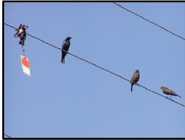
Figure 10-5. Birds perched next to spinning diverter.
