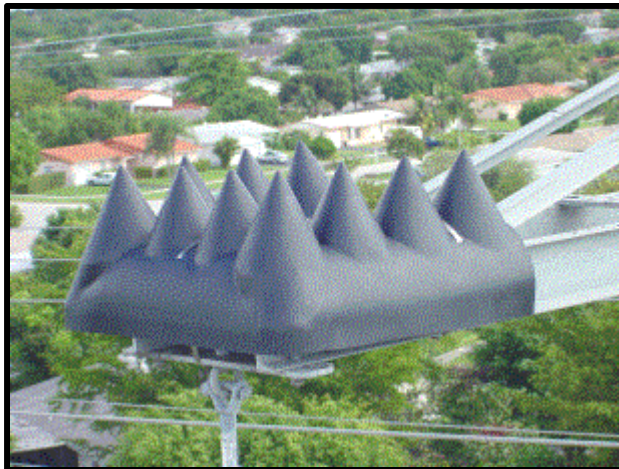
Figure 12-1. HDPE cones deployed on the arms of a lattice transmission structure (Zena Design).
