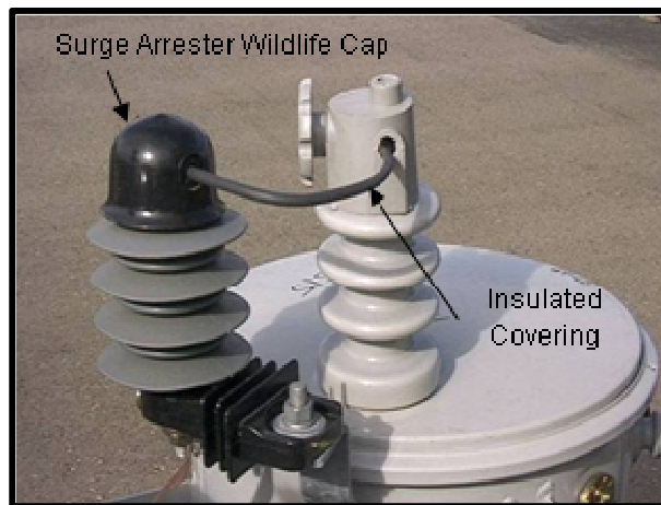
Figure 8-65. Transformer mounted surge arrester with wildlife cap.
