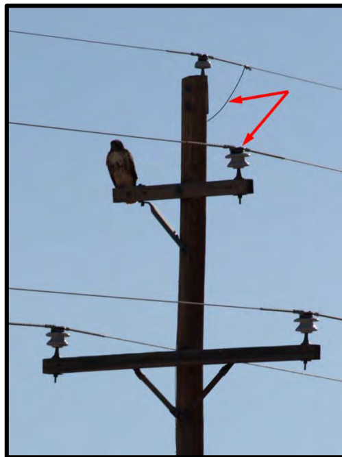
Figure 15-17. Groundwire should be covered at the top of pole.
