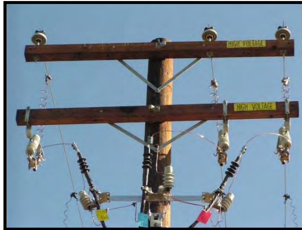
Figure 8-37. Unprotected riser pole.
