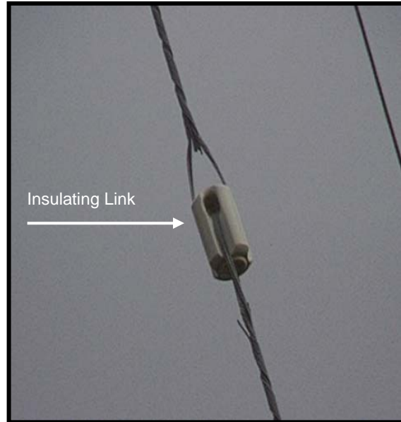
Figure 8-84. Insulating link to prevent a pathway to ground.
