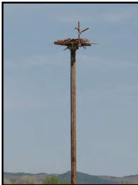
Figure 11-8 Nesting platform on a surrogate pole.
