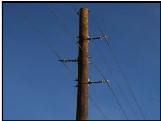
Figure 8-21. Vertical tangent unit (hardware is bonded).
