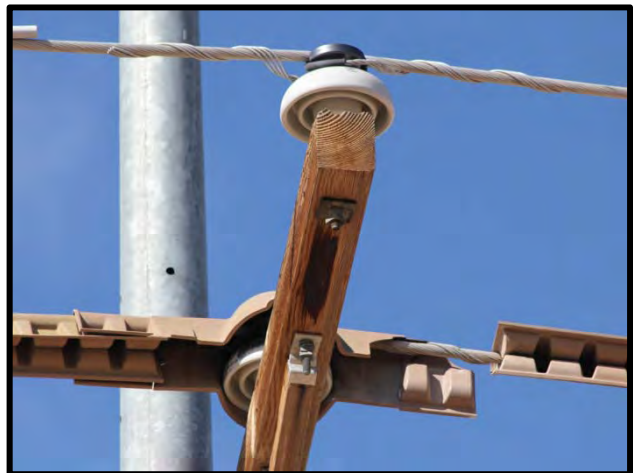
Figure 15-35. Close-up of conductor cover damage.
