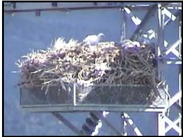
Figure 11-12. Eagle nesting platform on a transmission lattice tower.
