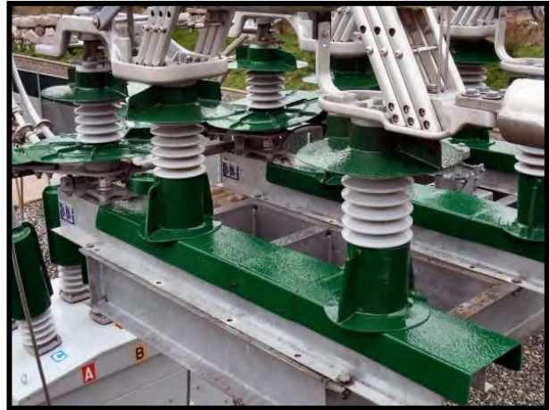
Figure 8-89. Switch with isolating plates.
