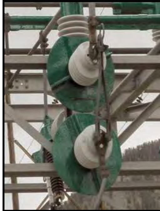
Figure 9-14. Switch barrier (Salisbury).
