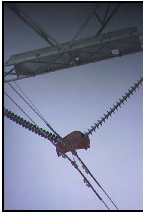
Figure 13-2. Fecal contamination insulated barrier (TE Connectivity).
