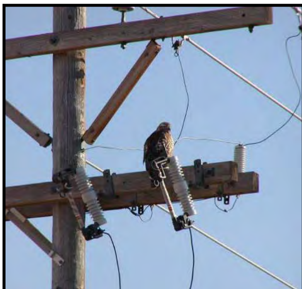
Figure 8-56. Hawk perched between unprotected cutouts and arresters.
