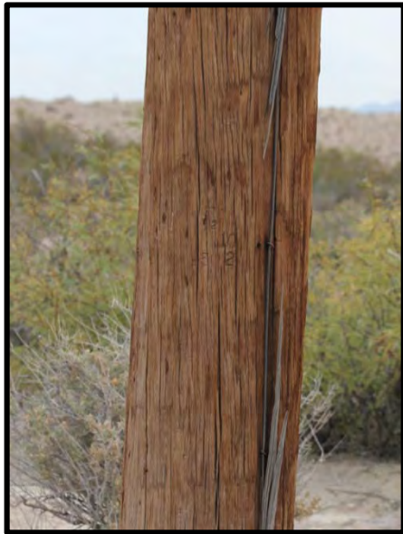
Figure 15-22. Deteriorating wooden molding for exposed groundwire.
