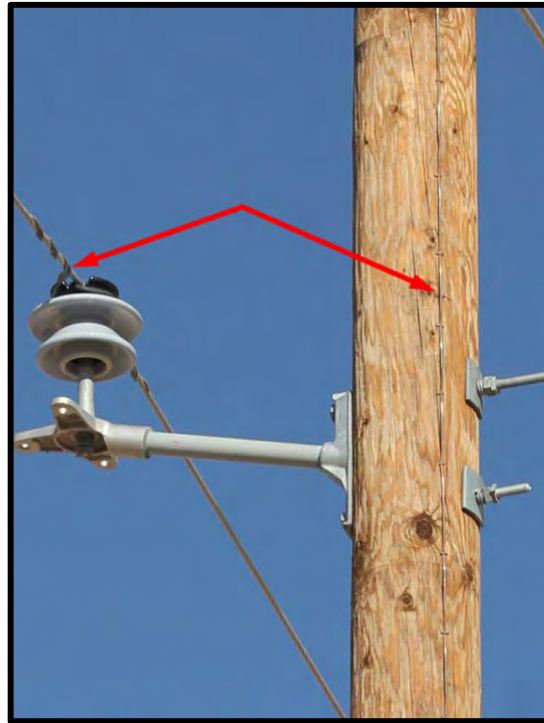
Figure 15-19. Close-up of exposed groundwire in proximity to conductor increasing electrocution risk for even smaller birds.
