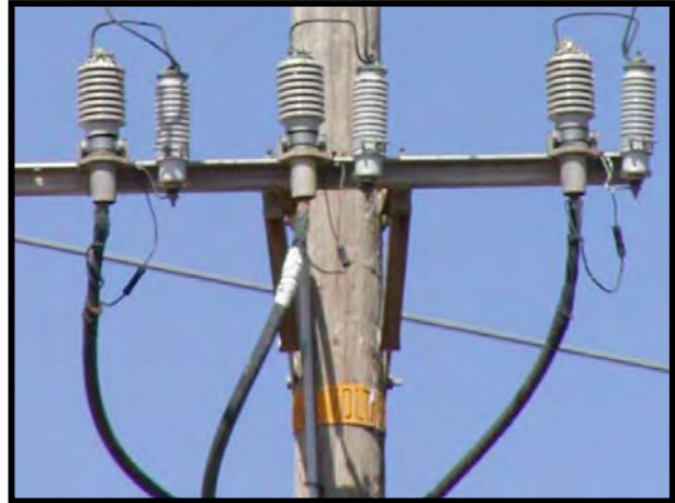
Figure 8-79. Three-phase grounded metal bracket with unprotected potheads/arresters and jumpers.
