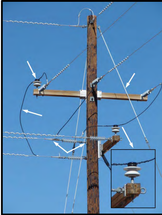
Figure 15-2. Double deadend with covered jumpers, covered pin insulators, and extension links on center phases.
