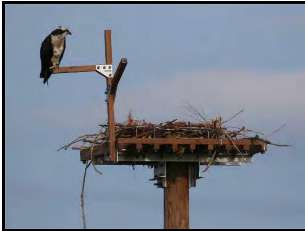
Figure 11-11. Osprey platform with an elevated perch on a surrogate pole.
