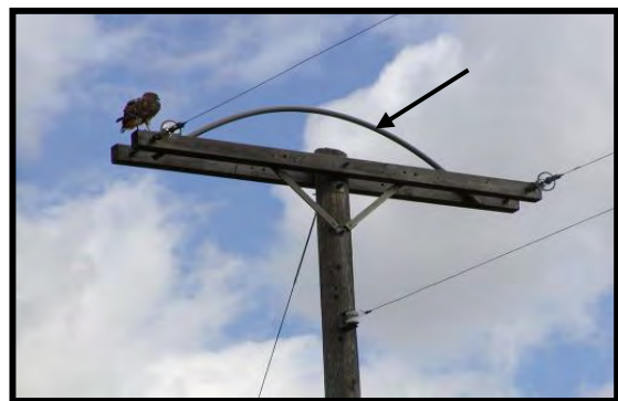
Figure 11-19. Stick deflector to keep nesting materials from attaching to the crossarm.
