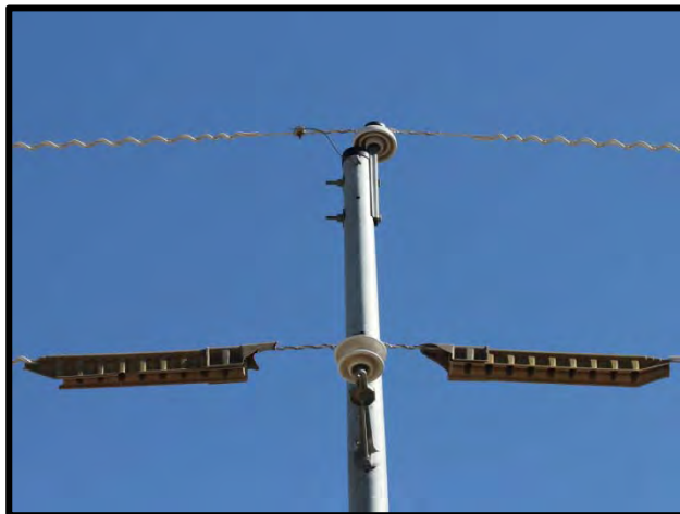
Figure 15-34. Conductor cover damage was recorded across WSMR.
