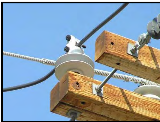
Figure 8-74. Covered jumper supported with a vice-top insulator (Hendrix).
