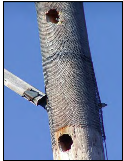
Figure 3-8. Woodpecker damage to a wood H-frame structure.
