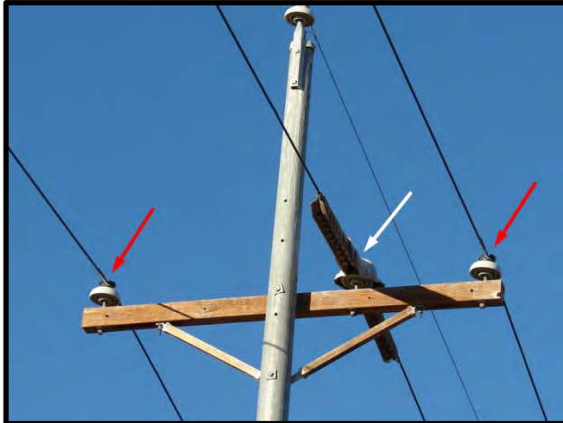
Figure 15-32. Steel structures require three conductor covers.
