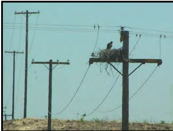
Figure 11-1. Problem Red-tailed Hawk nest on an unprotected distribution line.
