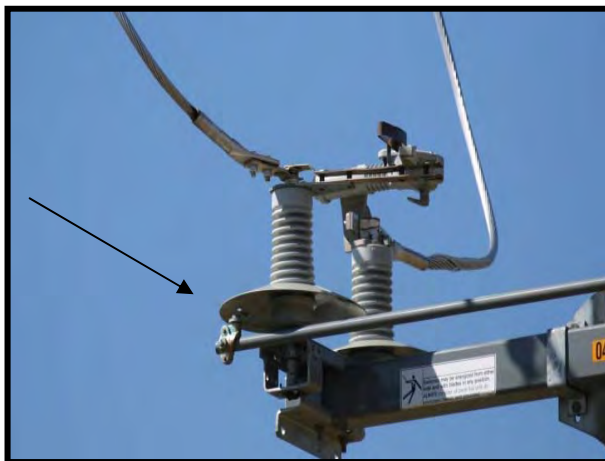
Figure 9-15. Switch with isolating plate.
