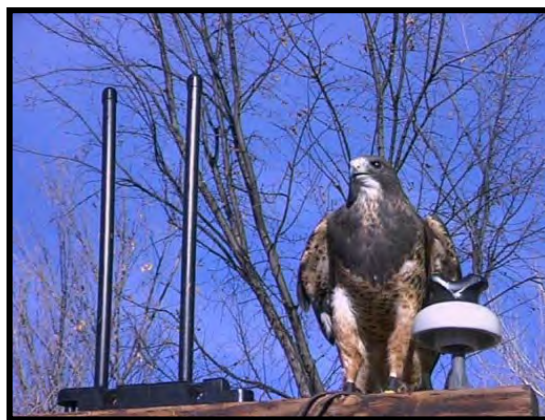
Figure 8-110. Example of improper use of bird spikes for perch management.
