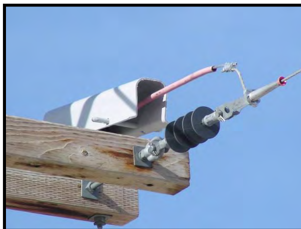
Figure 8-75. Covered jumper isolated with a pin cover.
