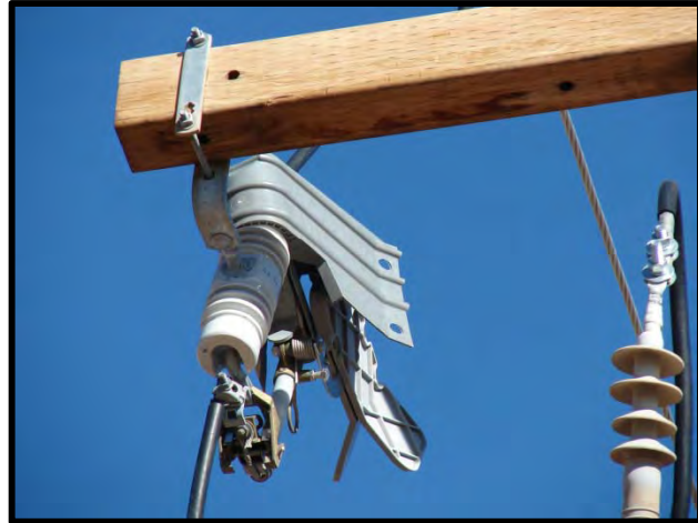
Figure 15-39. Misapplication of cutout cover over loadbreak cutout – appropriately designed cutout covers for loadbreak cutouts should be used.
