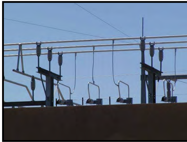
Figure 9-4. Substation bus supports for animal protection.
