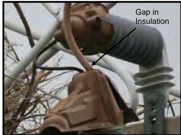
Figure 8-63. Cutout cover with gap between top of cover and bottom of jumper insulation.
