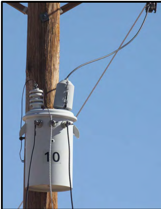
Figure 15-40. Single-phase with bushing cover installed too low on bushing sheds.
