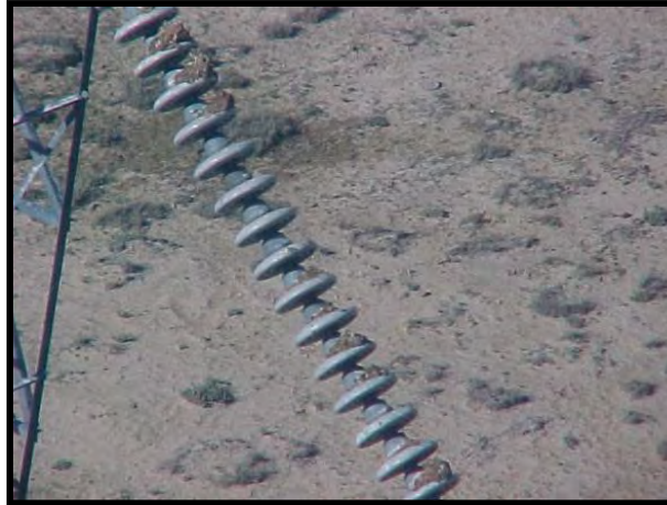
Figure 3-11. Accumulated avian excretion (bird pollution) on an insulator. Bird pollution can lead tracking faults, particularly on the underside of insulators where rain increases conductivity but does not wash insulators clean.
