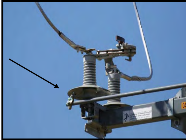
Figure 8-88. Switch with isolating plate.
