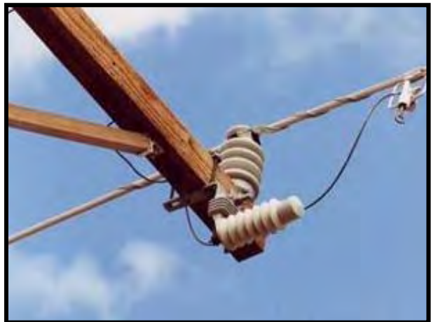
Figure 8-69. Underarm horizontally mounted surge arrester to reduce animal exposure.
