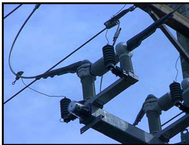
Figure 9-18. Switch with built-in animal protection (S&C Electric Company).
