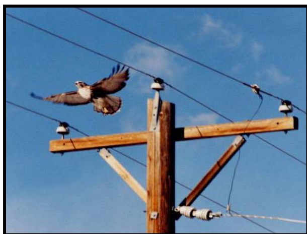
Figure 8-3. Typical tangent structure provides adequate separation (40 inches) for hawks.
