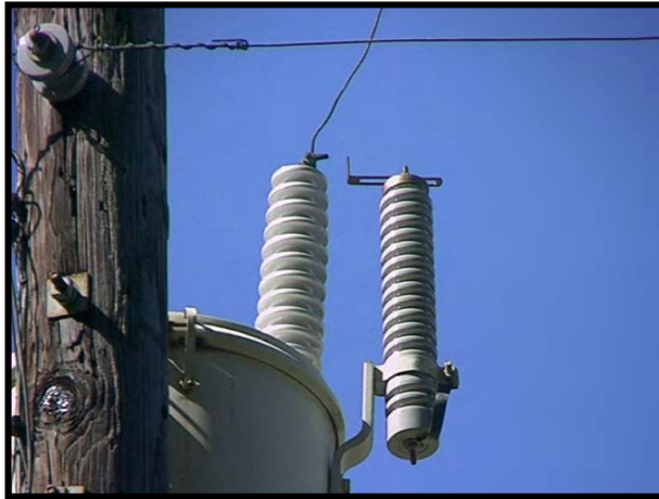
Figure 8-66. Transformer with gapped arrester.
