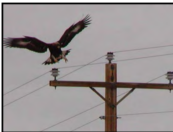
Figure 8-4. Typical tangent structure provides inadequate separation (60 inches) for eagles.
