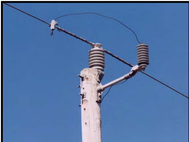
Figure 8-80. Single-phase ungrounded fiberglass bracket.
