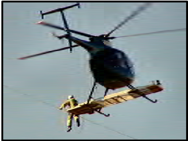
Figure 10-21. Installing SFDs with a helicopter.
