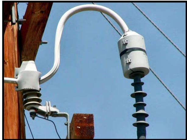
Figure 8-40. Protected riser pole (Hubbell Power Systems).
