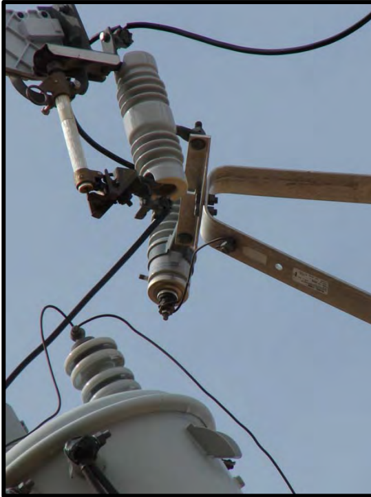
Figure 15-46. Grounded metal brackets supporting energized equipment present a high risk to even smaller birds.
