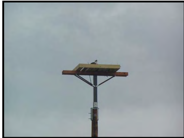
Figure 11-9. Osprey nesting on platform attached to pole-top extension.
