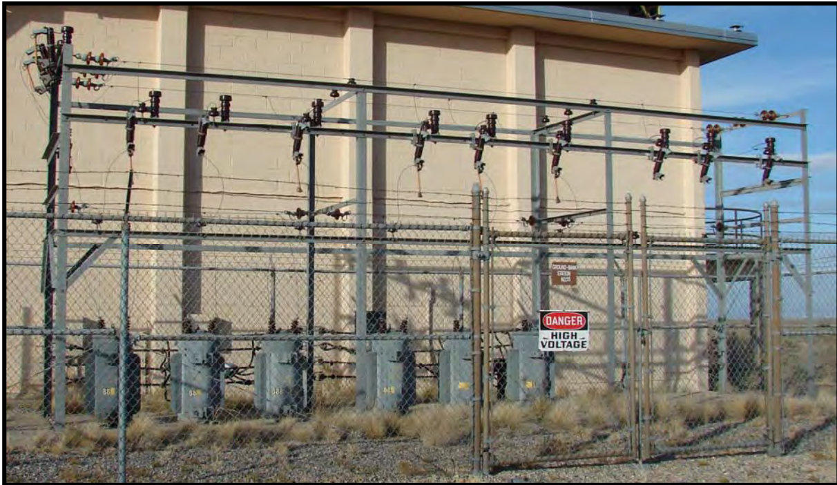
Figure 15-37. Ground Bank with newer equipment and very high-risk structure.
