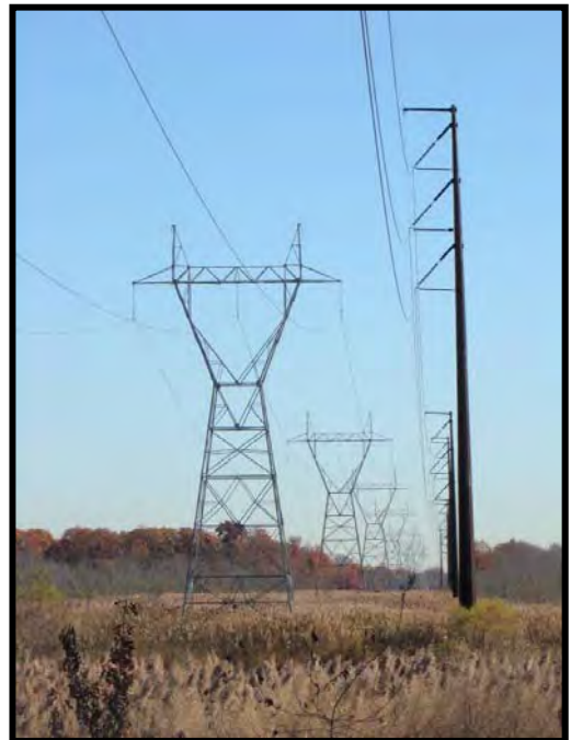
Figure 3-5. On the left, the wire orientation of the lattice structure in a horizontal configuration reduces the number of wire planes as compared to a vertical configuration on the right.
