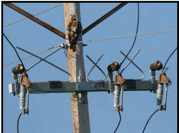
Figure 8-81. Three-phase ungrounded fiberglass bracket with protected cutouts/arresters and jumpers.
