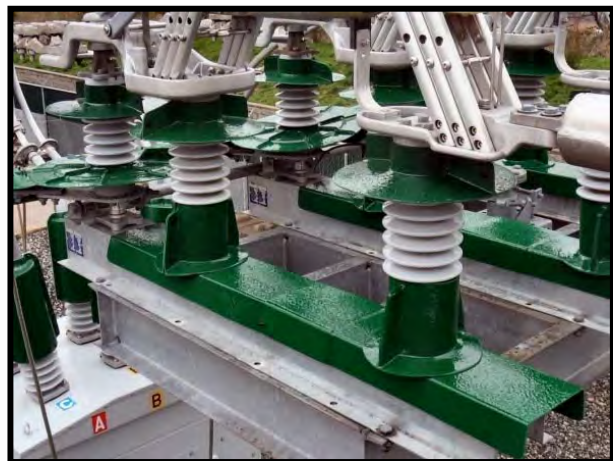
Figure 9-16. Switch with isolating plates (Salisbury).
