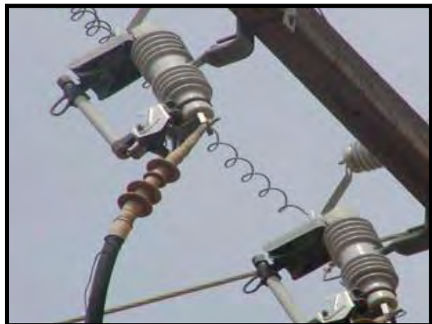
Figure 8-42. Riser mounted below cutouts.
