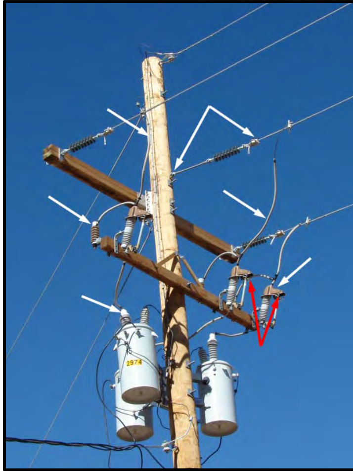
Figure 15-1. Equipment pole with good coverup and extension link in center phase. Cutout locking horns still exposed (see Figure 8-58).
