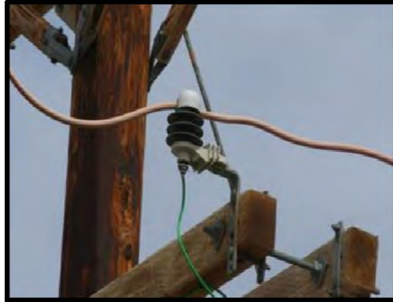
Figure 8-70. Surge arrester with cap and insulated groundwire.
