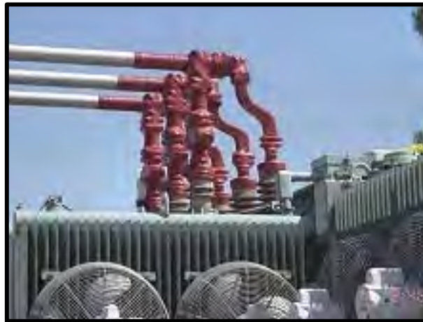
Figure 3-3. Substation fitted with insulation.
