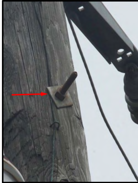
Figure 15-47. Groundwire bonding metal mounting bolt and grounding associated bracket.
