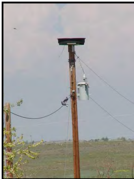
Figure 11-7. Nesting platform above a retrofitted single-phase pole.
