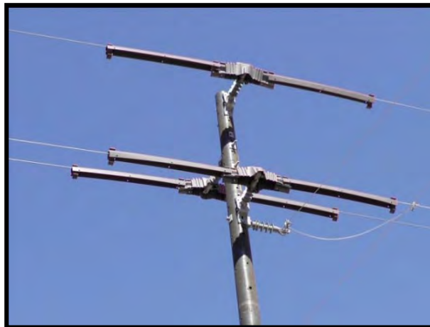
Figure 8-25. Horizontal post insulators covering each phase (TE Connectivity).
