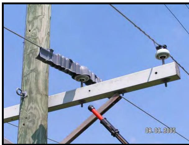
Figure 8-18. TE Connectivity conductor cover.
