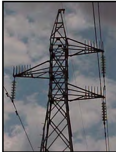
Figure 12-2. HDPE spikes deployed on the arms of a lattice transmission structure (Mission Engineering).
