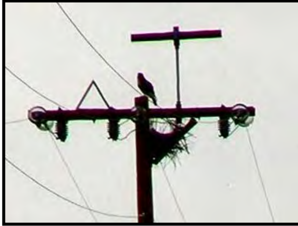
Figure 8-94. Raptor perching below an elevated perch.
