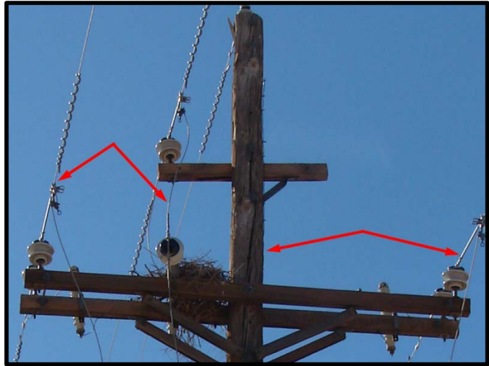
Figure 15-16. Older tangent configuration C1-2 OHN with one single and one double crossarm – cover groundwire and center phase jumper wire.
