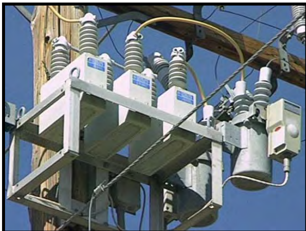
Figure 8-52. Capacitor bank factory-ordered with animal protection.
