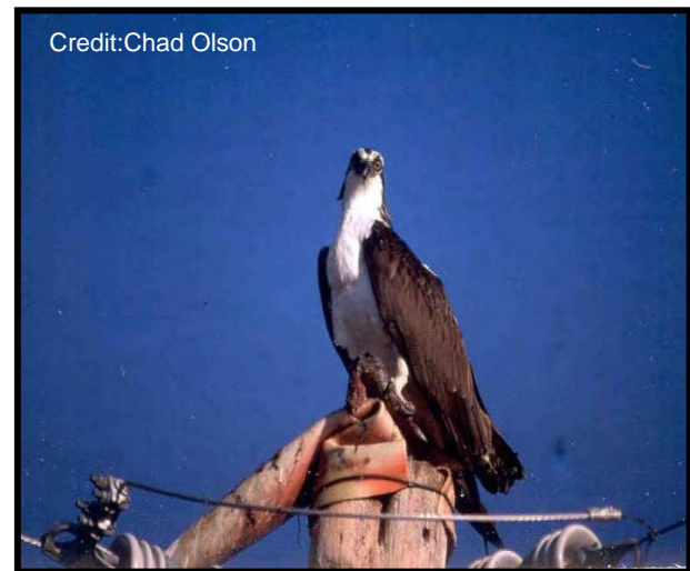
Figure 8-103. Inappropriate use of a traffic cone as a perch discourager.
