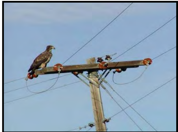
Figure 8-29. Three-phase double deadend with jumpers passing under the crossarms (bird-friendly).
