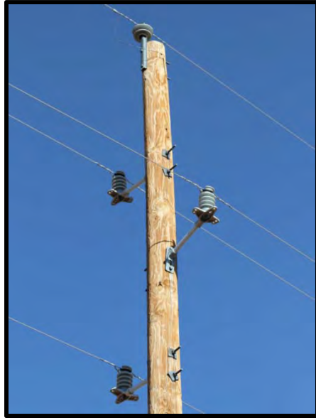
Figure 15-20. Common three-phase vertical configuration at WSMR.
