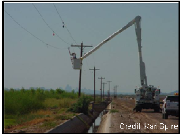
Figure 10-7. Flapper installation.
