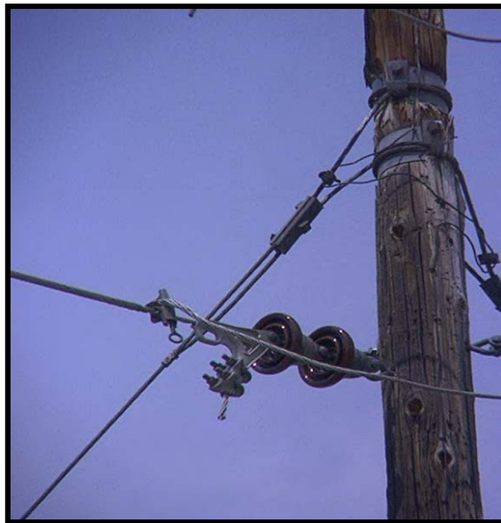
Figure 8-85. Guy wires attached to grounded pole bands.
