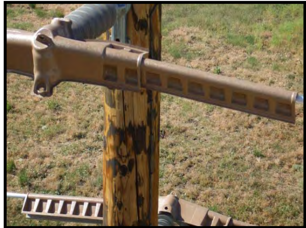
Figure 8-24. Covering each phase with a conductor cover (Kaddas).
