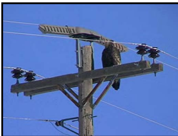
Figure 8-17. Kaddas conductor cover.
