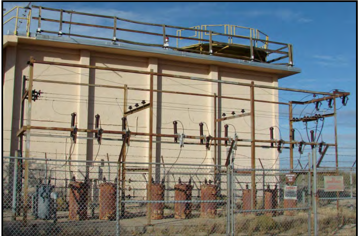
Figure 15-36. Ground Bank with older equipment, but still energized. Very high-risk structure.
