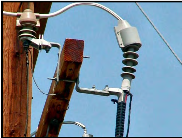
Figure 8-39. Protected riser pole (Salisbury).
