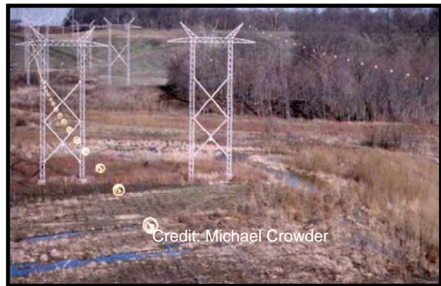
Figure 10-14. SFDs installed at 20-foot intervals in Indiana.
