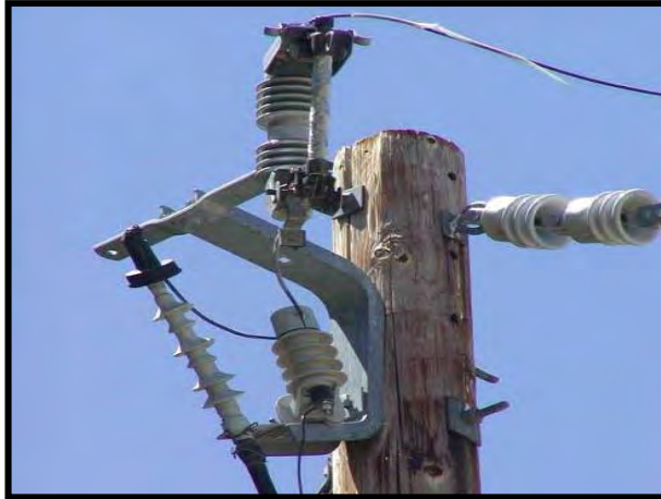
Figure 8-78. Single-phase grounded metal bracket with unprotected cutout/arrester.
