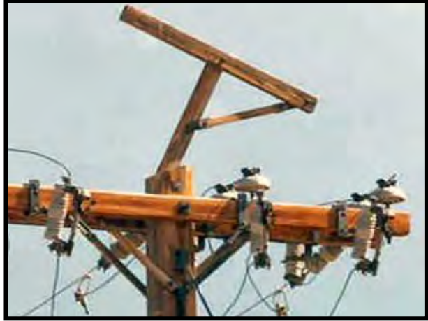
Figure 8-95. Improperly installed elevated perch and unprotected pole.
