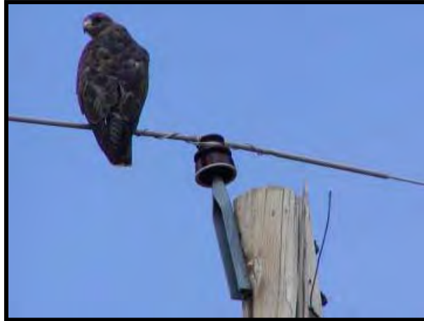
Figure 8-76. Exposed pole-top groundwire
