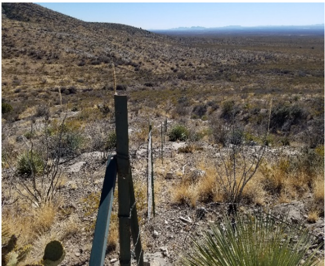
Photograph 5: Example 4-strand Wire Fence with T-Posts
