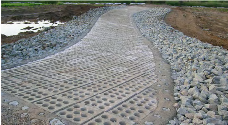
Figure 2-2. Interlocking Concrete Block Crossing with Riprap Apron
