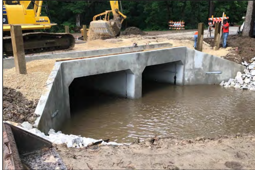
Figure 2.5 Concrete Box Culvert Installation
