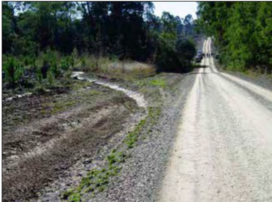
Figure 2.7. Turnout Collecting and Discharging Water from a Roadside Ditch
