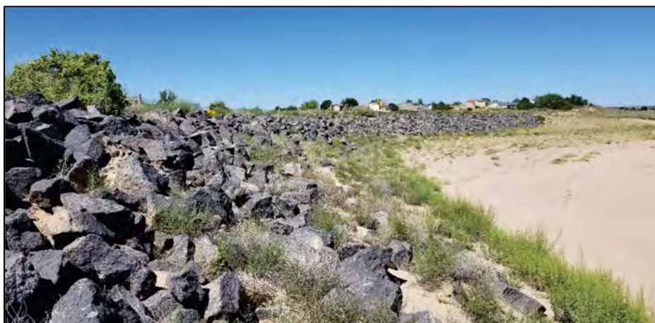
Figure 2-6 Vegetated Riprap Bank Protection
