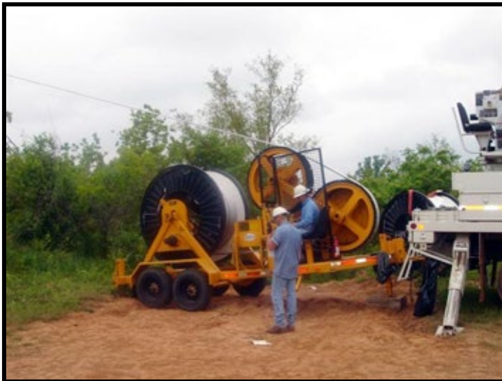
Figure 2-3 Tensioner Equipment within Temporary Work Area
