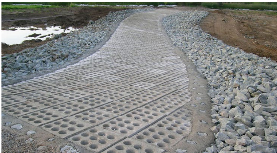
Figure 2-2. Interlocking Concrete Block Crossing with Riprap Apron
