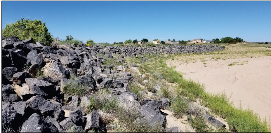
Figure 2-6 Vegetated Riprap Bank Protection
