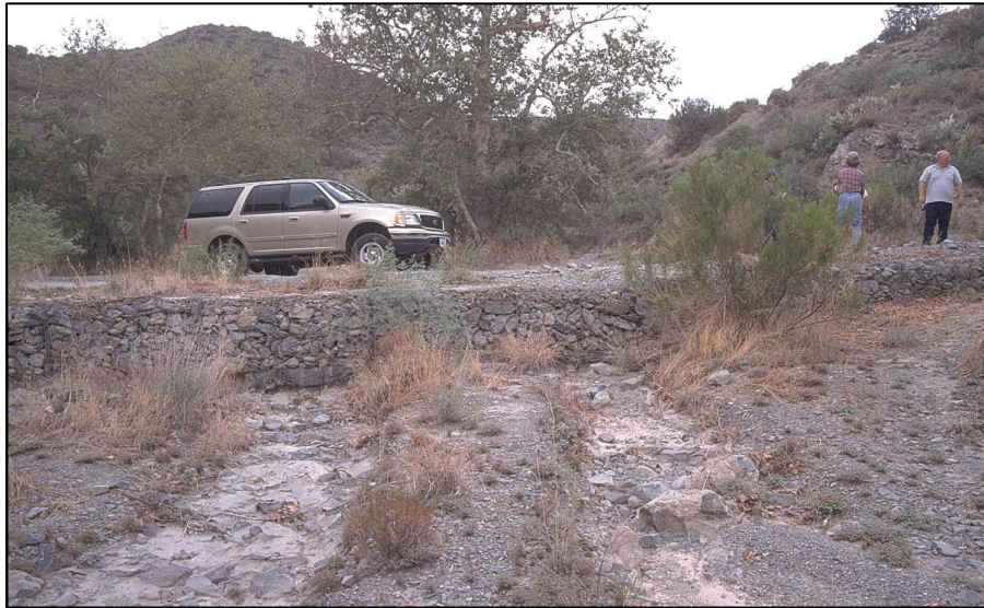
3 4 Figure 2-3. Gabion Ford View from Downstream
