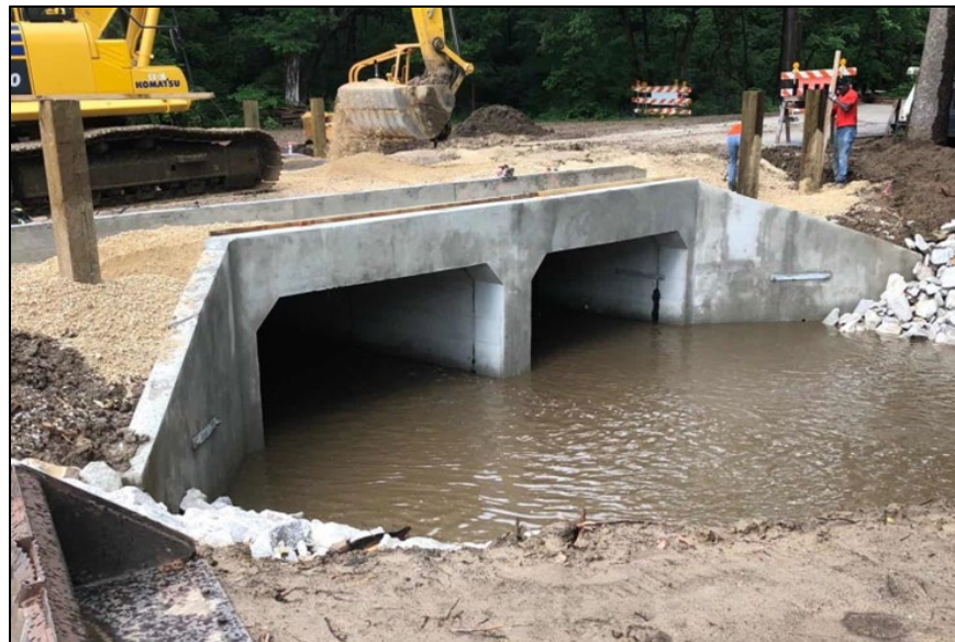
Figure 2.5 Concrete Box Culvert Installation
