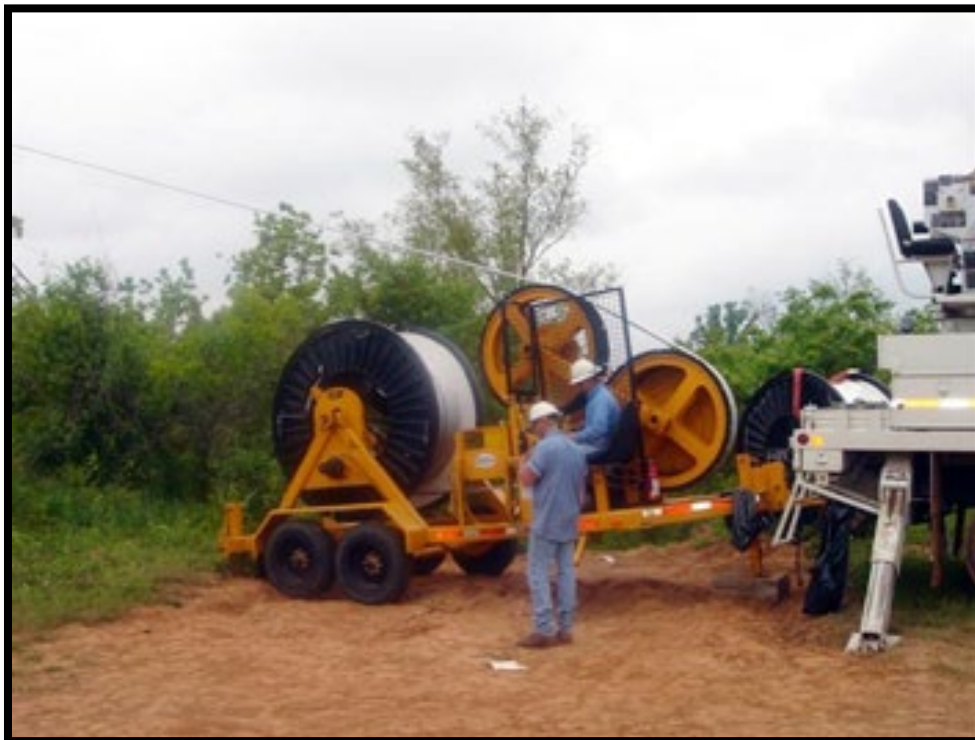
Figure 2-3 Tensioner Equipment within Temporary Work Area
