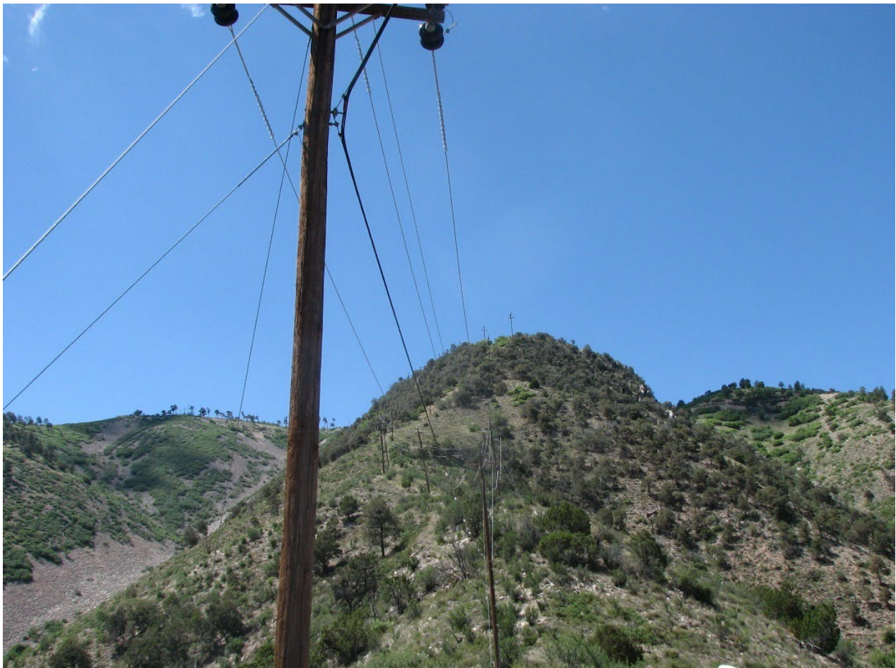
Figure 1-2 Steep Slope along Route
