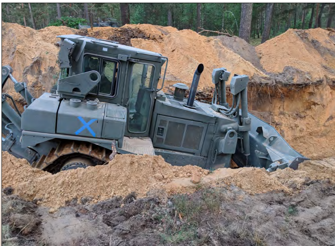
A Soldier uses a bulldozer to dig an antivehicular ditch during engagement area development.
