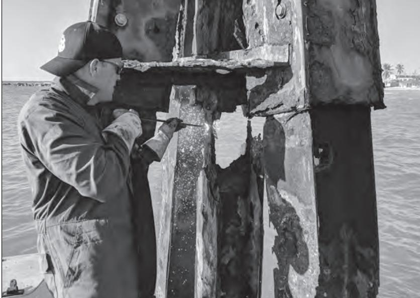
**An Army master diver uses a BROCO exothermic cutting rod to detach I beams on the surface, Andros Island, Bahamas.**
