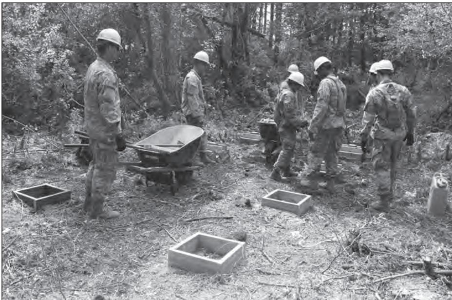
**Exposed substructure during construction of the elevated walkway at Murray Creek**
