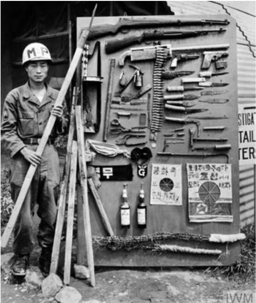
Figure 7.2. Sergeant Chang Myong-oh, a Republic of Korea military policeman, displays weapons found in Prisoner Compound No. 72, Koje-do. EPWs made the knives and spear heads from the steel supports of their shoes, the sharp daggers from oil drum metal, and spears from tent poles. Photo courtesy of the US Army.
