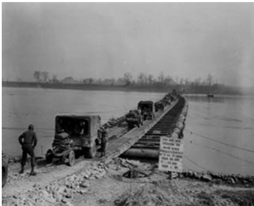
Figure 5.3. Traffic crossing a treadway bridge over the Rhine River south of Wesel. Photo courtesy of US Army Engineer School History Office.
