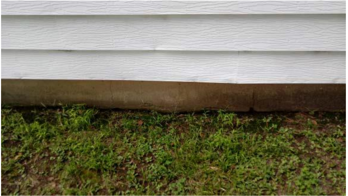
Figure 1. Foundation cracks due to differential settling.
