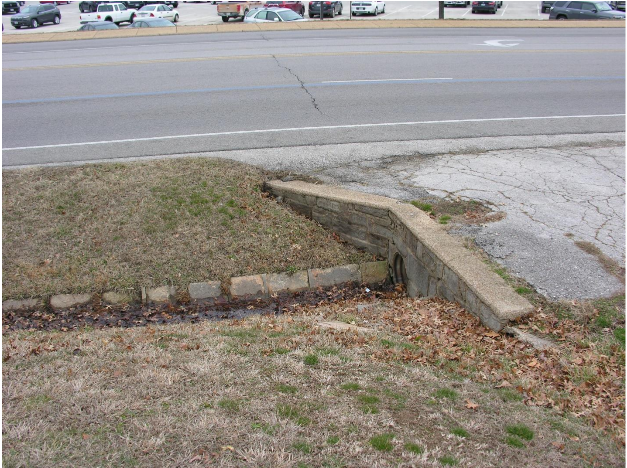
Figure 8. POW stonework culvert and headwall.
