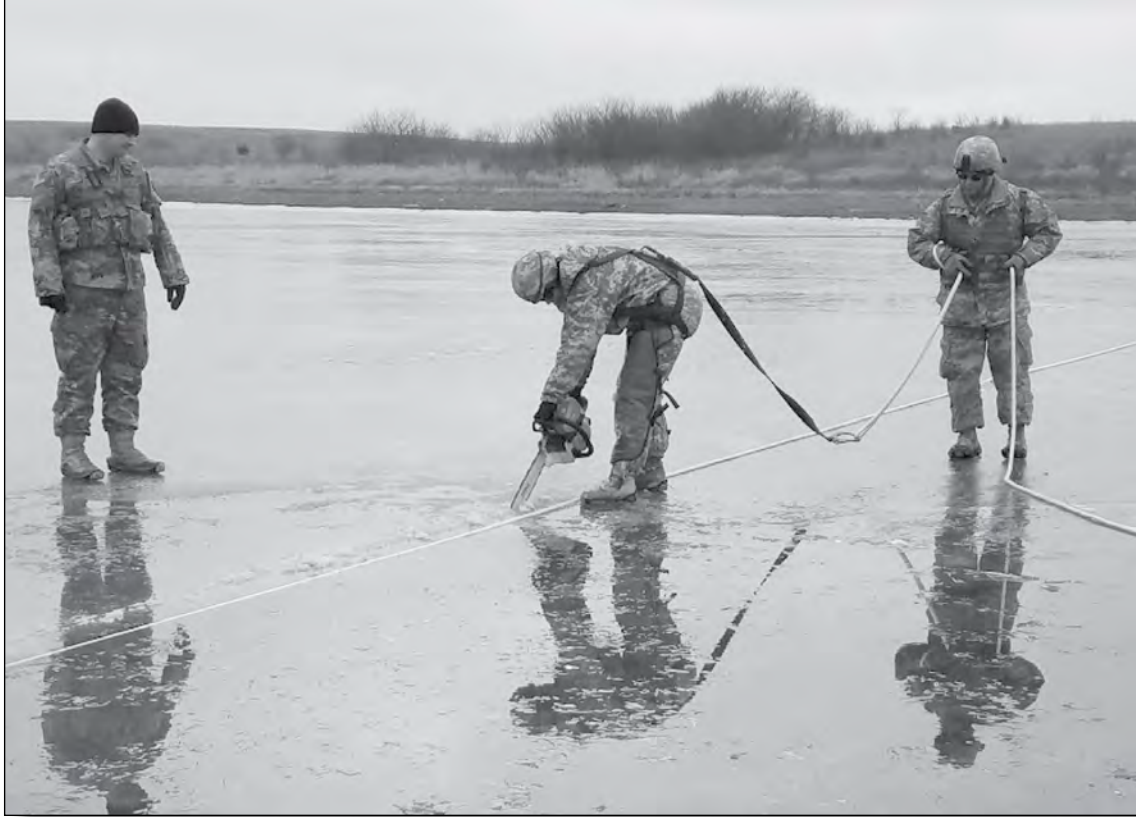
A 143th MRBC Soldier and safety guides scroll a line in the ice with a chainsaw in an attempt to break the ice away from the main body.
