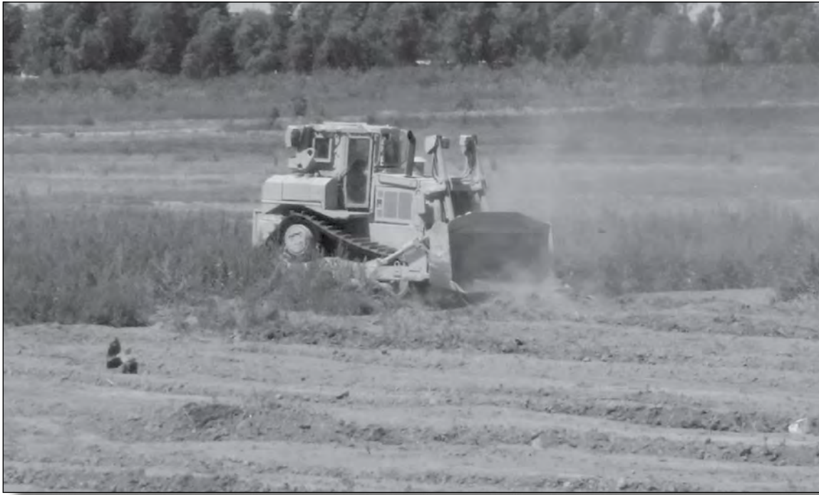
Dozing operations conducted by equipment operators at a TAA in Mosul, Iraq. The equipment operators immediately began constructing the TAA once the area was deliberately cleared.
