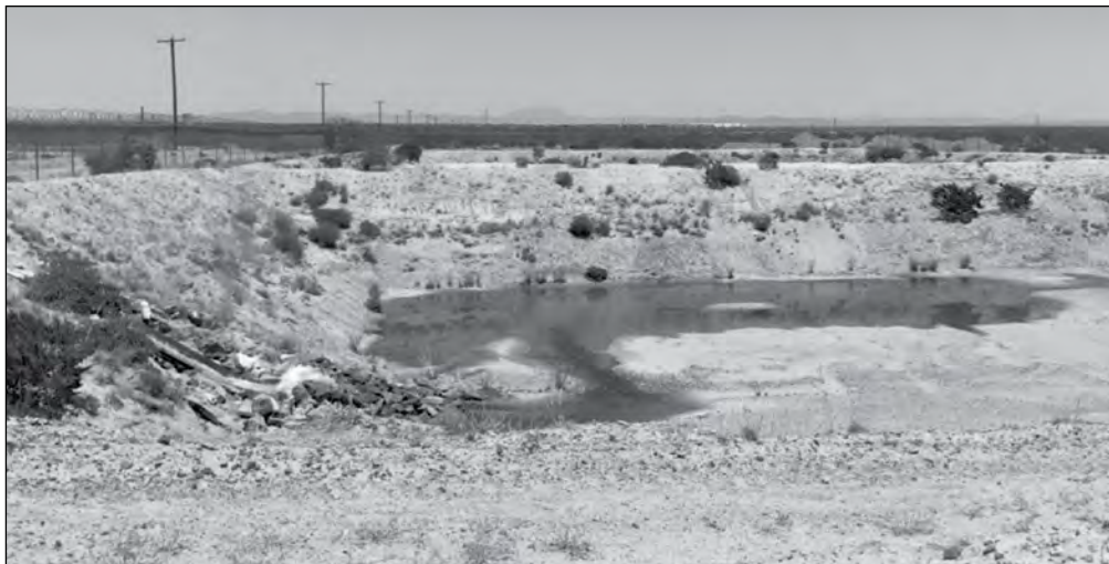
Figure 1. A 0.3-acre infiltration basin in El Paso, Texas, where a continuous inflow of 300 gallons per minute was observed for 36 hours in June 2017.
