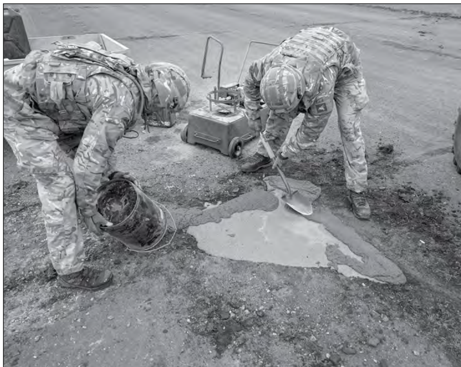
Paratroopers assigned to the 23 Parachute Engineer Regiment utilize LARP assets to fill potholes in the runway.
