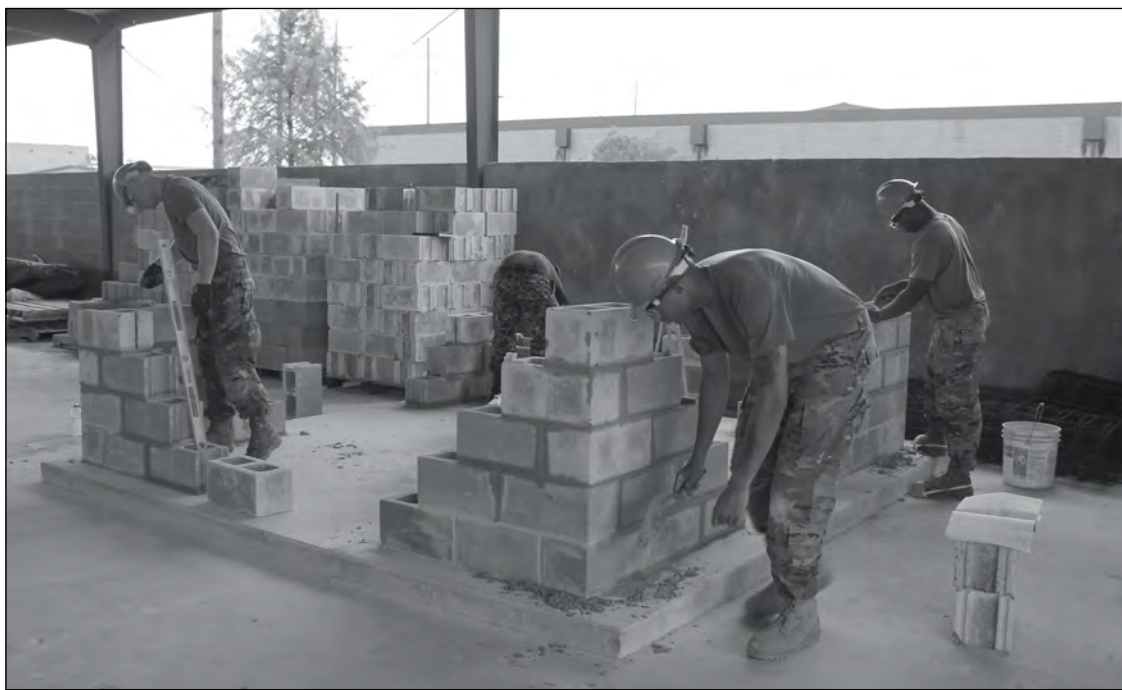
Soldiers and Sailors practice their corner lead concrete masonry skills at the Naval Construction Training Center at Gulfport, Mississippi.
