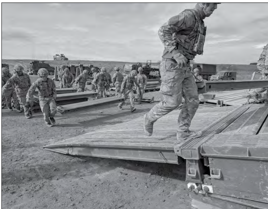
Paratroopers assigned to the 23 Parachute Engineer Regiment rush to complete a medium girder bridge to allow friendly armored reinforcements access to the drop zone.
