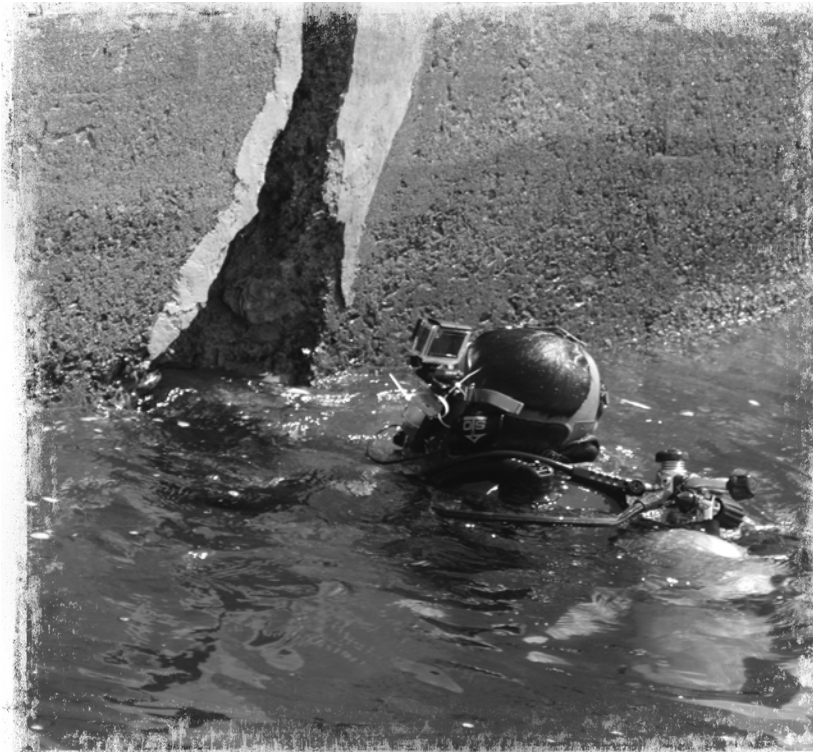
A diver surveys and records video of a critical structural deficiency in a concrete seawall during inspections.
