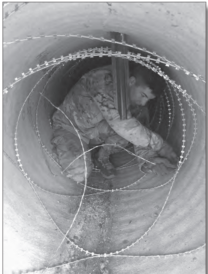
A Soldier builds a culvert denial system in Laredo, Texas.
