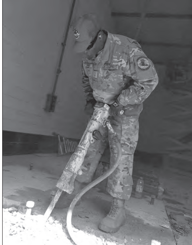
An Airman demolishes a concrete pad during deployment to the Republic of Korea.
