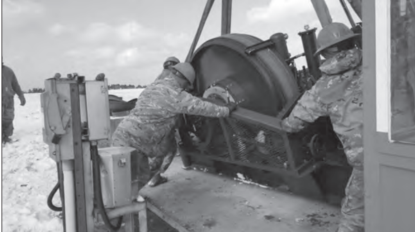
Airmen assist in reinstalling a barrier-arresting kit at Kunsan Airbase, Korea.
