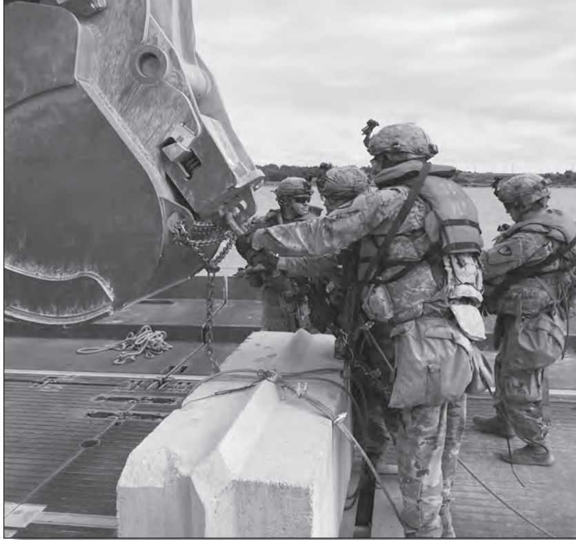
A cabling team moves a chain from the HYEX to the deadman anchor system.
