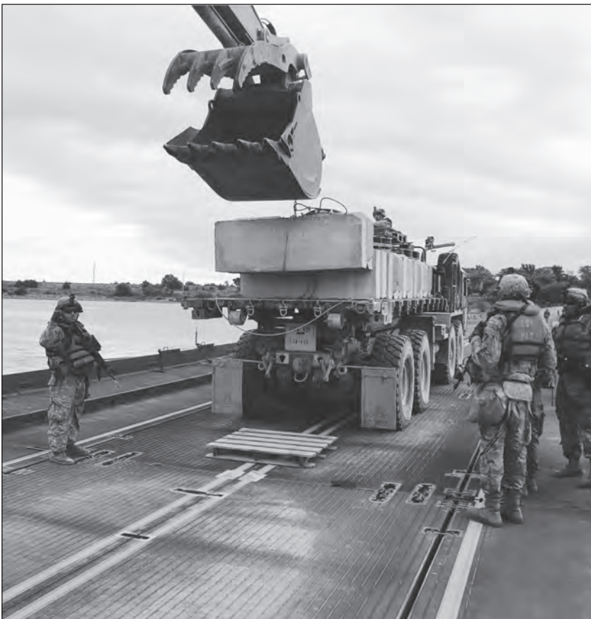
A Soldier guides a HYEX operator loading a deadman anchor onto a pallet.
