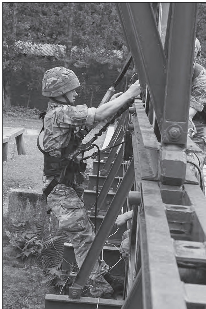
A trainee installs bridge demolitions.
