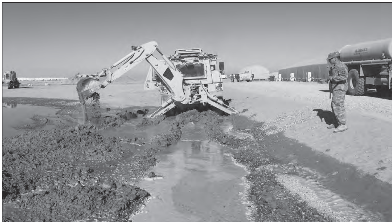
Engineers expand a drainage ditch to alleviate flooding after a heavy rainfall.
