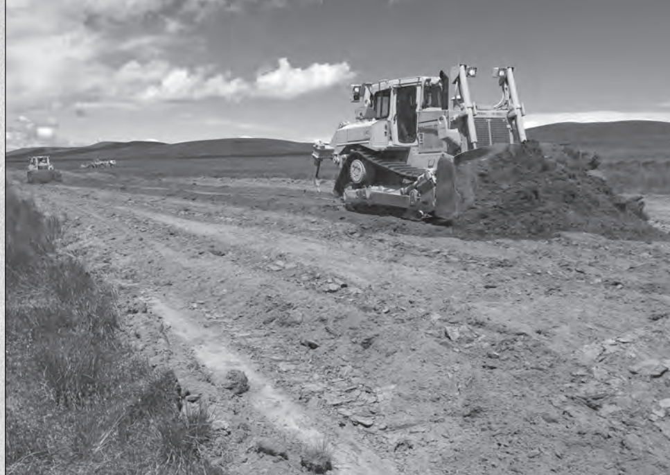
Soldiers from the 557th Engineer Construction Company use D7R bulldozers to rough grade the airstrip for a tactical unmanned aerial surveillance launch and recovery site at the Yakima Training Center in eastern Washington.
