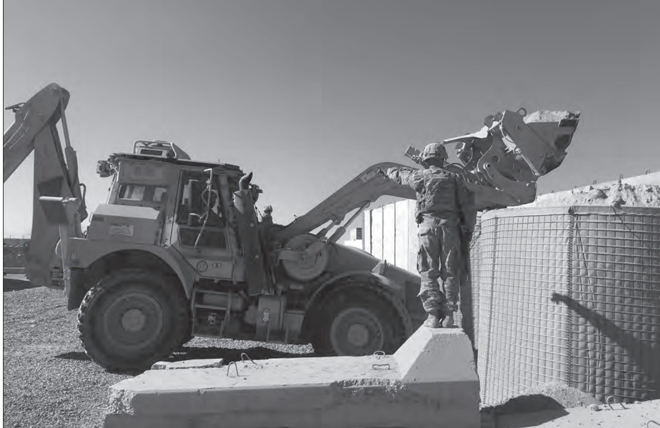
Soldiers fill HESCO® bastions to improve base force protection.
