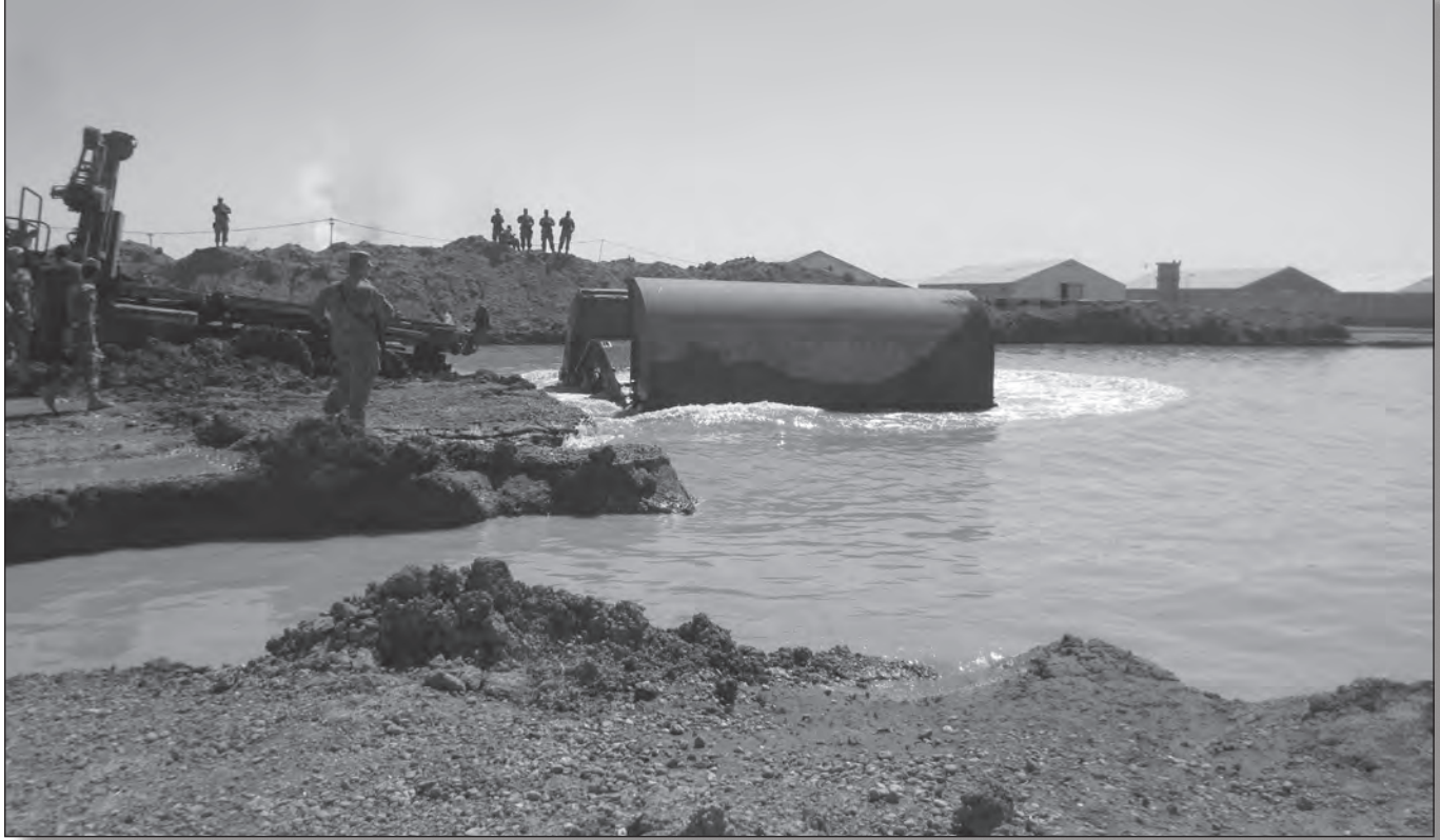
Iraqi soldiers deploy a bay for an improved ribbon bridge.
