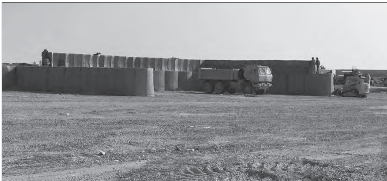
U.S. engineers construct an ammunition holding area.
