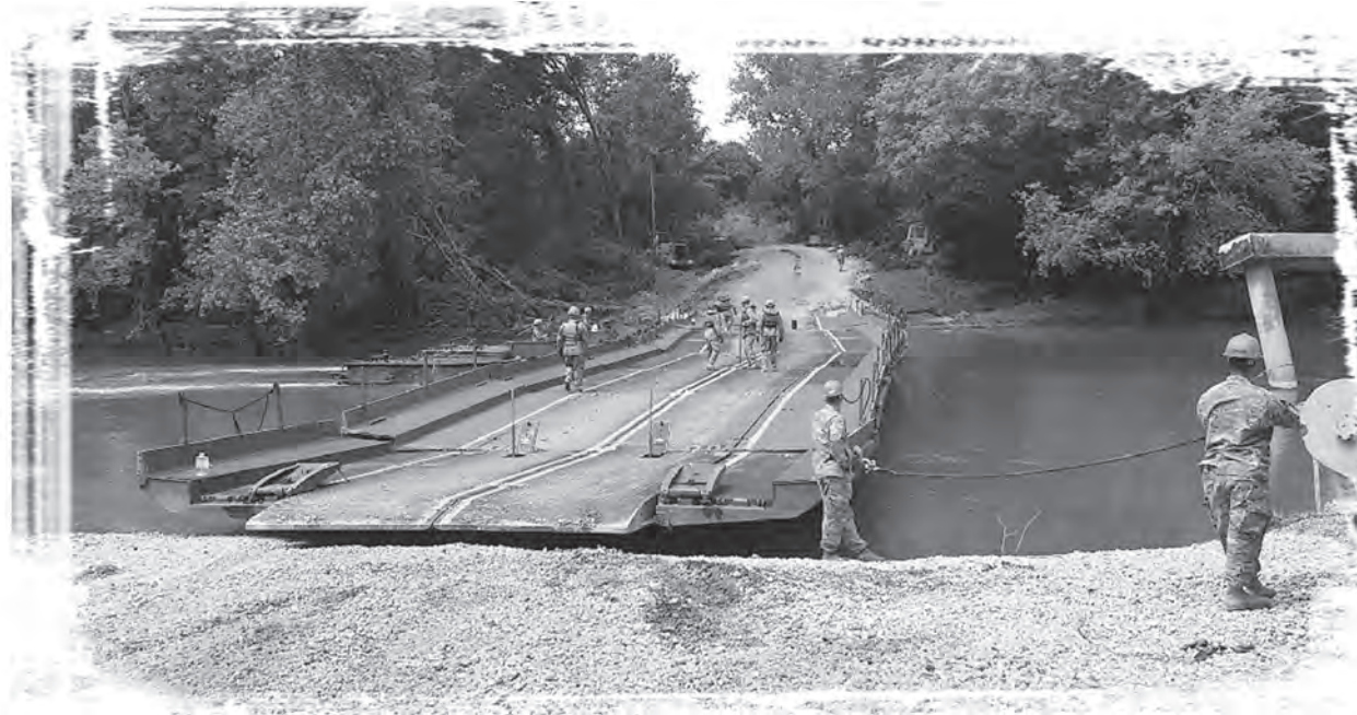
An improved ribbon bridge construction project over the Big Piney River provides an opportunity for adaptive application of program-of-instruction training.
