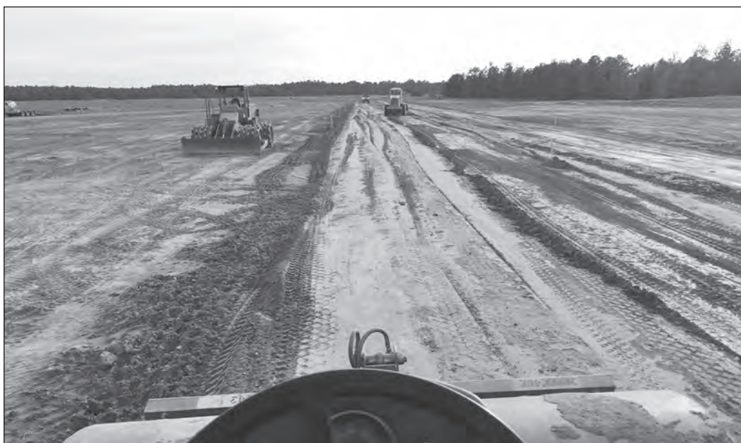
A high-speed compactor and vibratory roller compact the base course.
