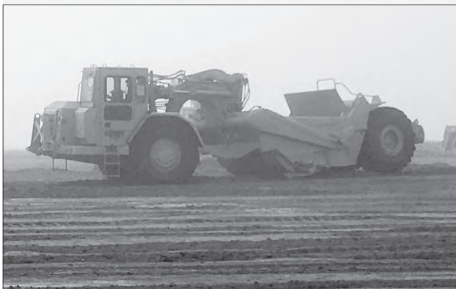
A scraper emplaces a 3-inch lift of dirt for the base course.
