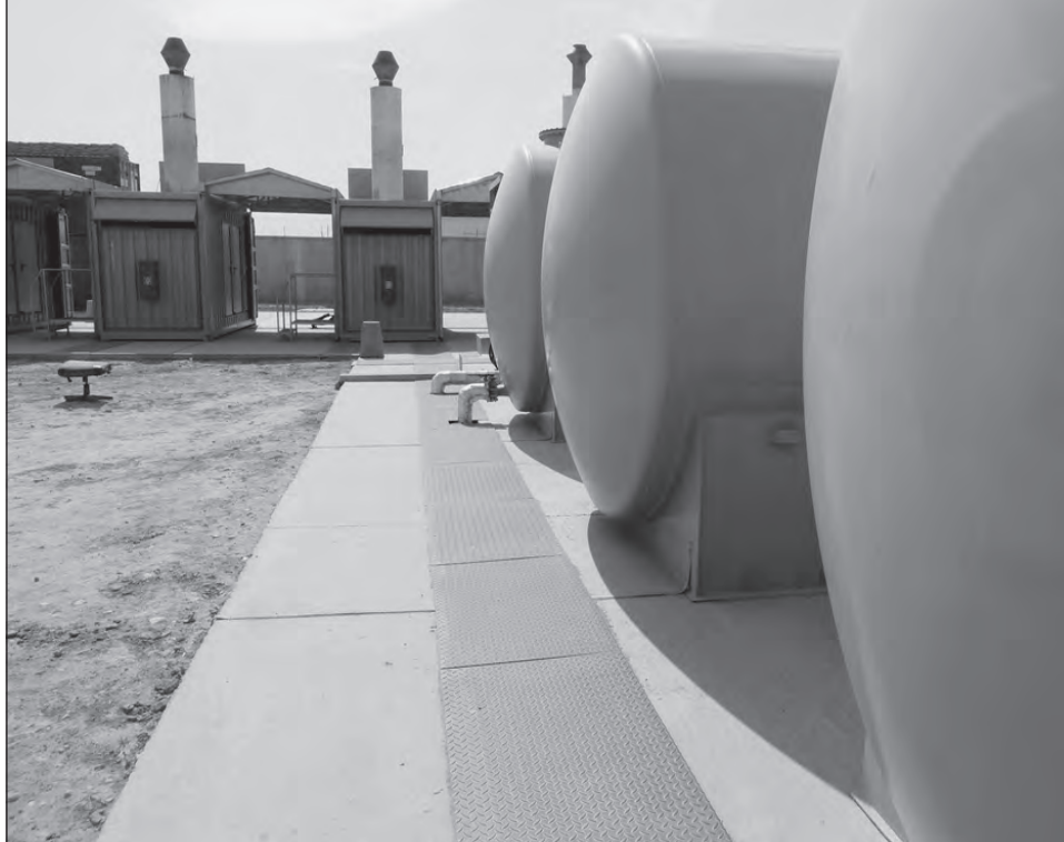
German forces at Mazar-e-Sharif maintain environmentally safe, double-walled fuel storage tanks for the generators that power the installation.
