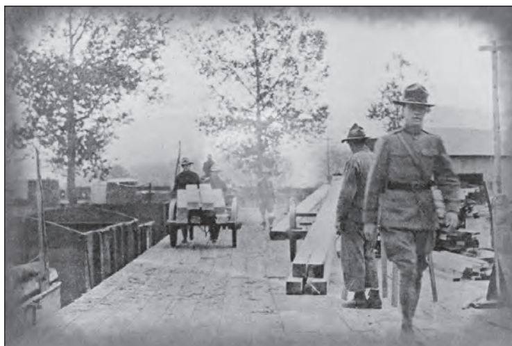
Loading some of the many thousands of ties made by the 20th Engineer Regiment mills for AEF operations in France.
