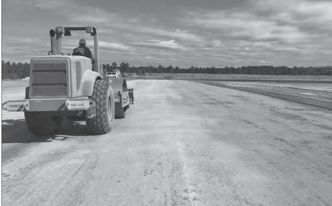
The select grade is compacted.
