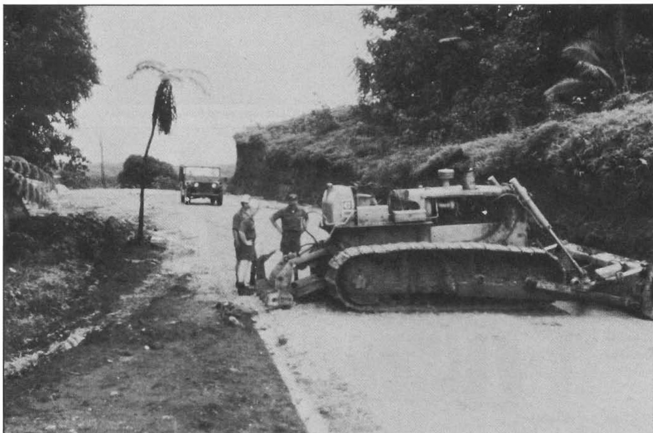
An old D6 dozer from a Ponapean agriculture station was used for borrowing operations.
