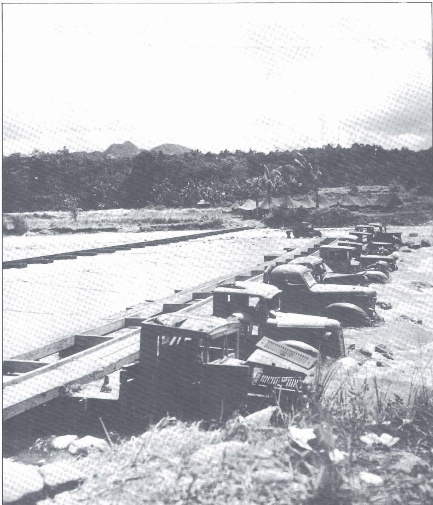
An improvised wooden treadway bridge is supported by the beds of old trucks placed in the stream. Cables on the upstream side were used to hold the vehicles in place. A floating footbridge is upstream from the vehicle bridge. (Photo taken somewhere in the Pacific during World War II.)
