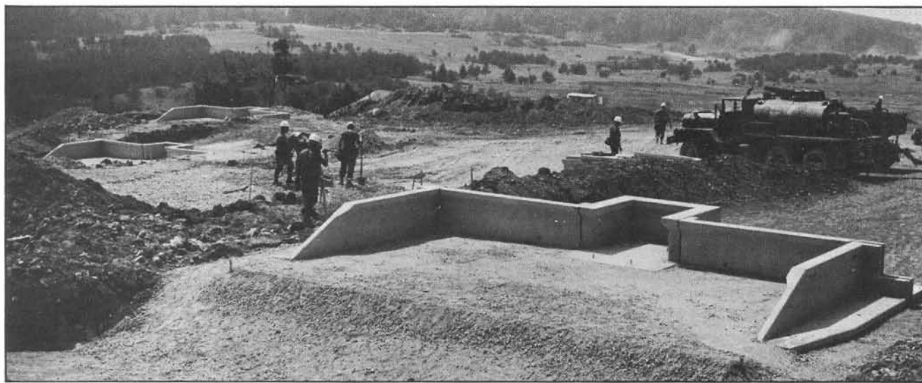
Construction underway on vehicle target pits at Range 42, Grafenwoehr Training Area, Germany.
