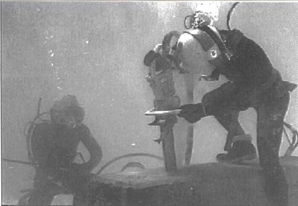
A diver cuts concrete with the hydraulic chain saw, a component of the Underwater Construction Set.
