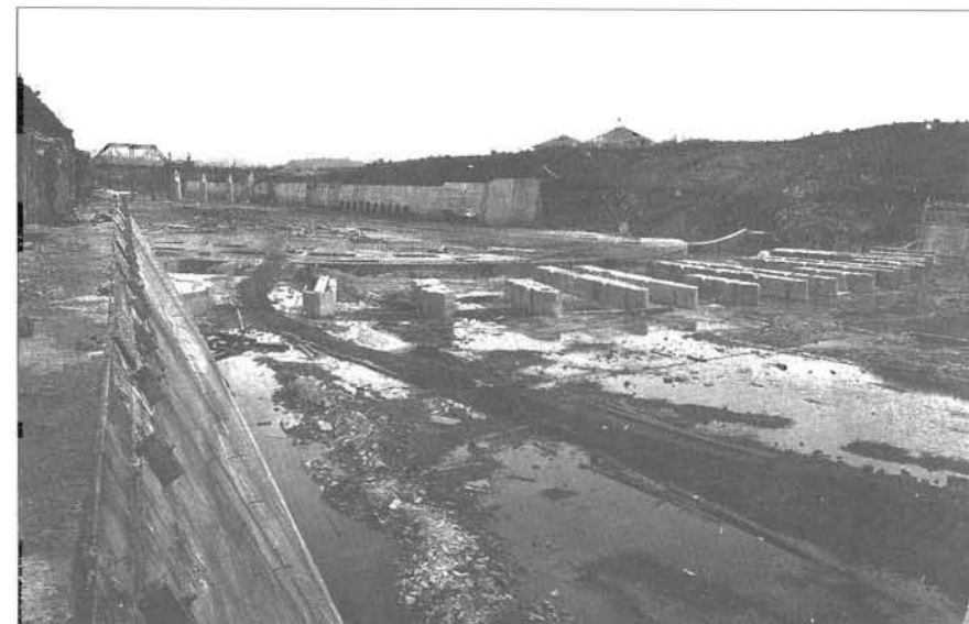
The spillway, looking north from the west wall. Foundations for valve and cofferdam piers are in the foreground.
