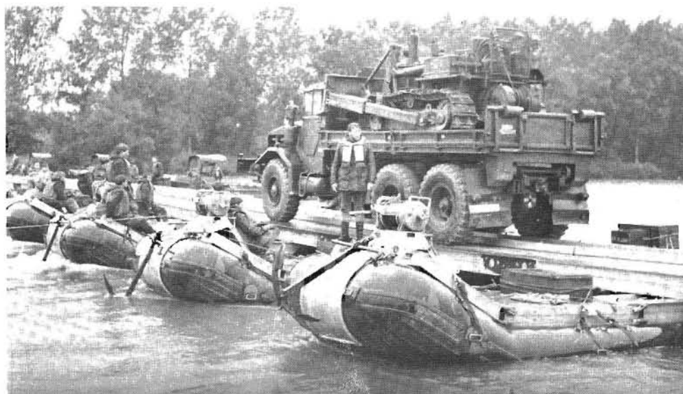
Troops load test a Bundeswehr pneumatic float bridge constructed by personnel of Pionierbataillon 12 and D Company, 9th Engineer Battalion on the Danau River.
