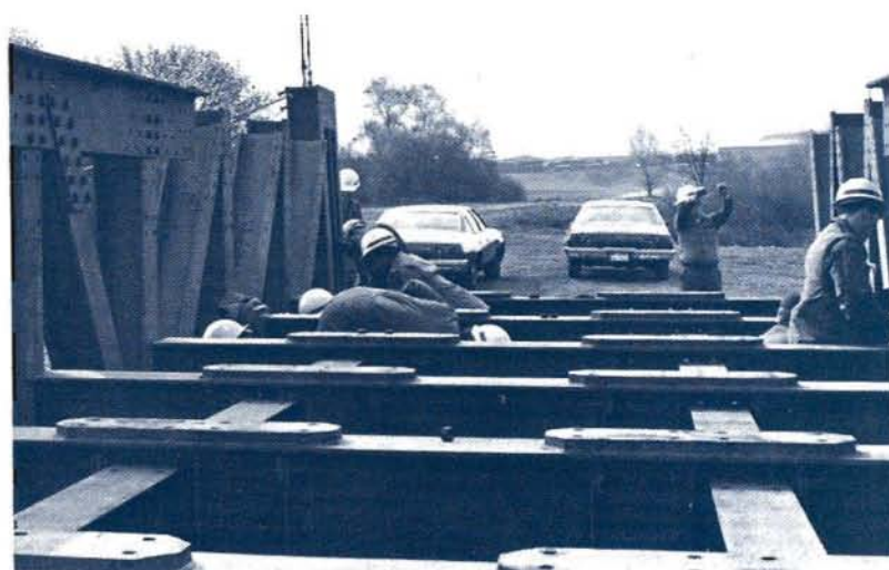
Troops assemble unit construction railway bridge.
