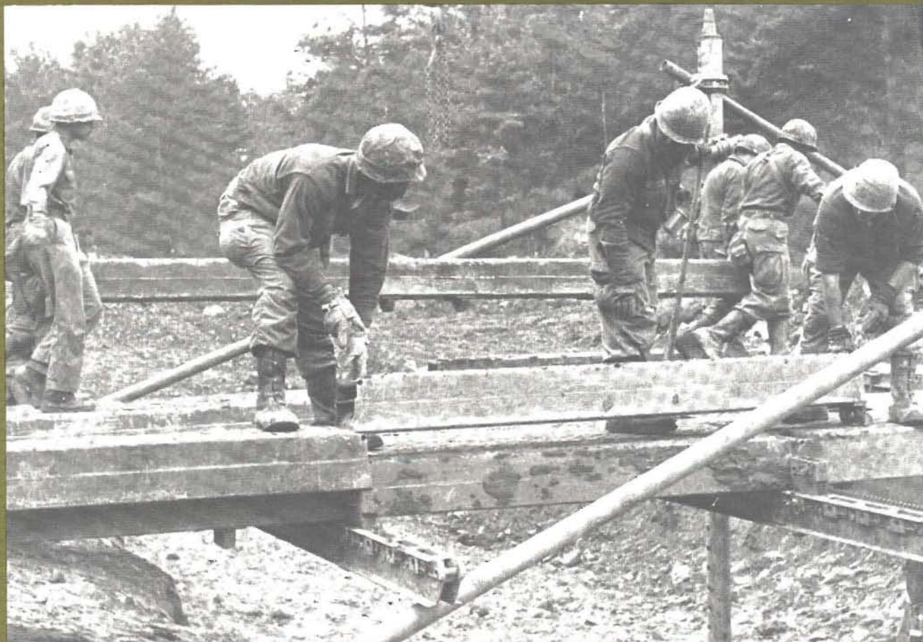
Constructing M4T6 Deck Balk Bridge with intermediate support
