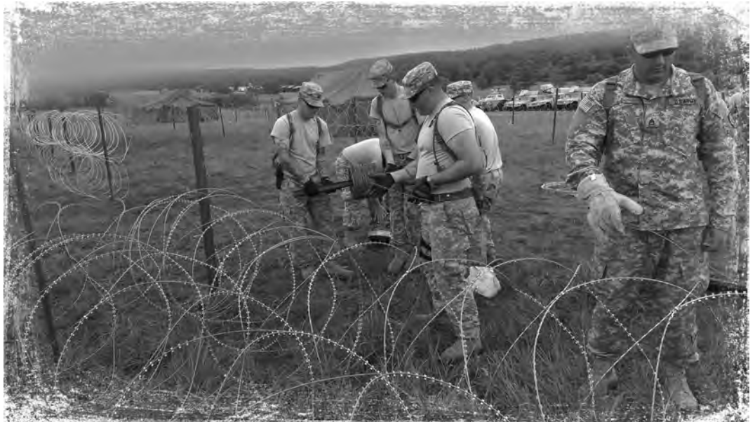
Soldiers of the 988th Military Police Company construct the perimeter of the DHA.
