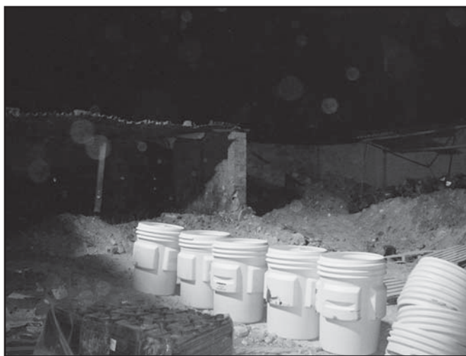
Overpack containers ready to be filled
