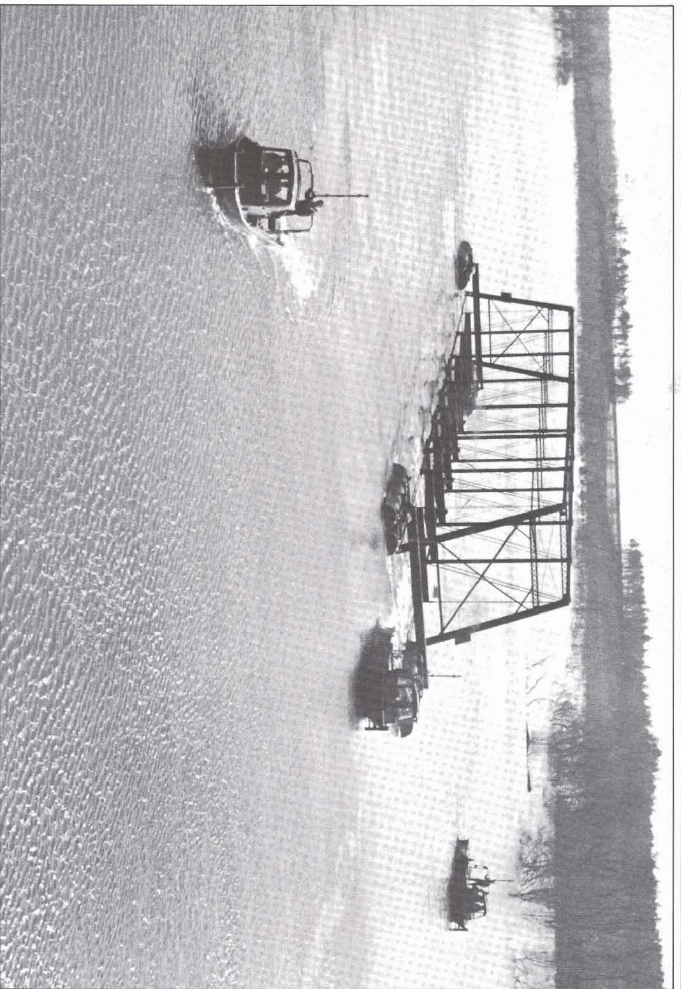
Endangered by rising waters, the Blackwell Bridge is towed to its new location. The bridge is a historic example of the American bridge pin connection system. Bridge-movement operations were conducted by the 3rd Engineer Bn., Ft. Stewart, while the new bridge site was prepared by Ft. Stewart's 92nd Engineer Bn. The operation was directed by the Corps' Savannah District.
