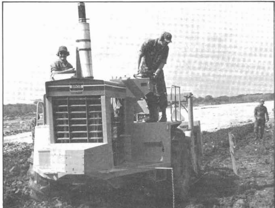
A leased Rototiller is used to reduce soil particle size before lime application. Several days of tilling were required because of the soil's high in-place water content.
