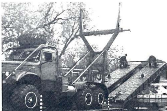
Truck-mounted multiple span bridge (TMM)
