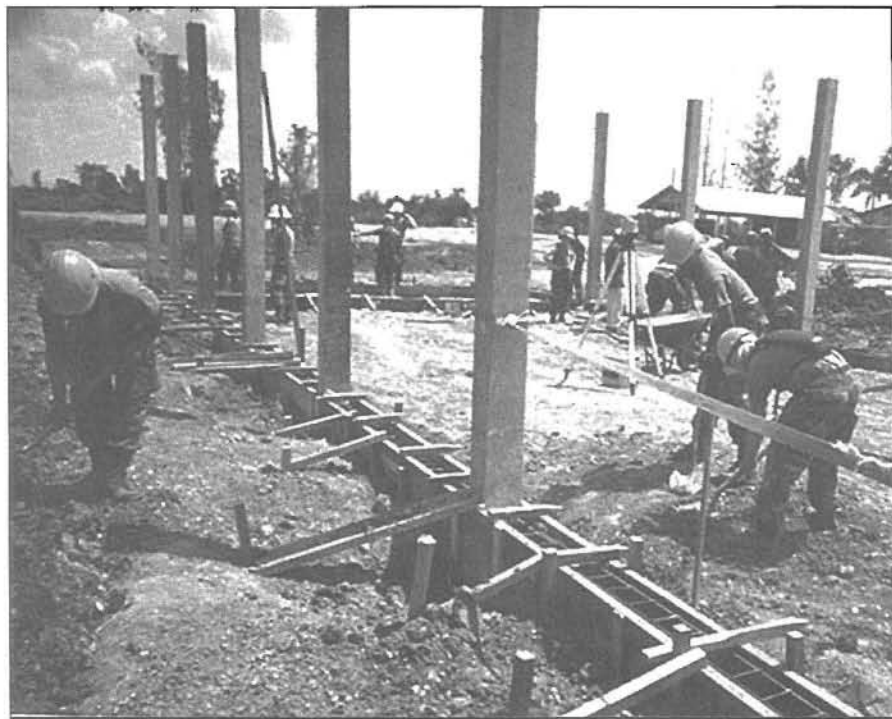
Soldiers from the 864th Engineer Battalion construct the foundation system for a multipurpose building in Thailand.
