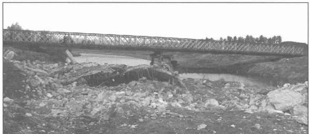
Figure 3. A bypass bridge made of DMS-65 structure elements with a continuous beam of 33 meters + 33 meters in length and access spans of 3 meters in length. The remaining parts of a destroyed bridge of 59 meters in length (Pilce town on the Nysa Klodzka River) are shown in the foreground.
