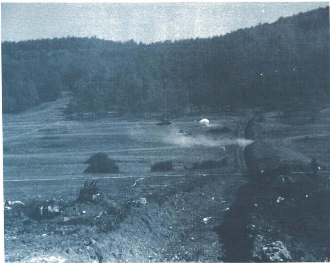
RECTANGULAR ANTI-TANK DITCH are better than triangular in clayey soil, but tougher to counter attack across.
