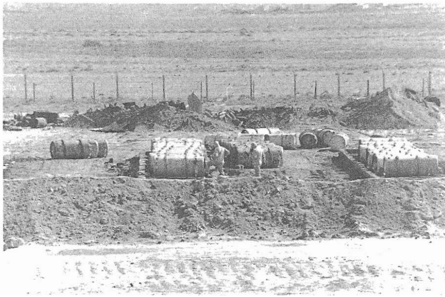
United Nations EOD personnel prepare to set charges for the explosive venting of mustard one-ton containers.
