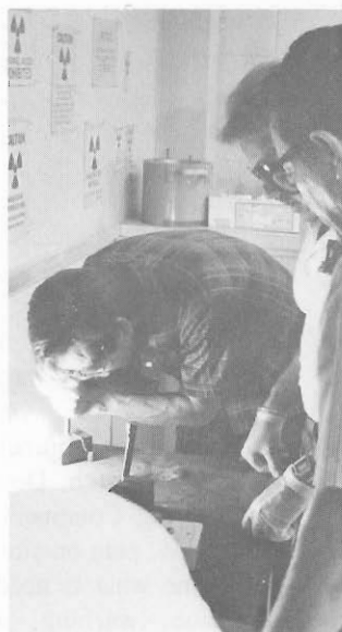
Above, SSG Ward reads a dosimeter prior to certifying it with the UDM-2 calibrator, above right. Right, a student zeros a dosimeter.
