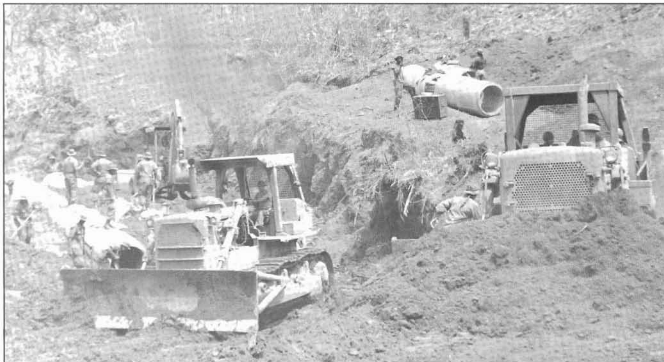
The 135th Engineer Group, Missouri National Guard, installs culvert on the Azuero Peninsula in Panama. Here, two bulldozers cut into the harsh jungle terrain.
