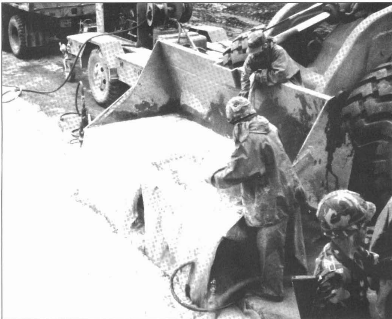
Testing in a realistic environment reveals the combat heavy TOE is inadequate for rapid airfield damage repair. Here, engineers from the 961st combat heavy place cement. The TOE modifications being considered by the Directorate of Combat Developments would overcome current problems with quality, equipment, and time.
