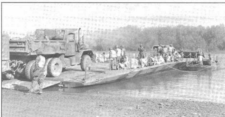
Working against swift current, Arkansas National Guardsmen complete this 800-foot bridge in 36 minutes.
