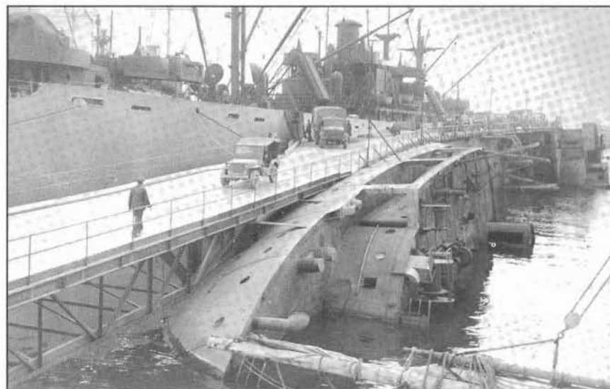
Engineer ingenuity converted sunken ships into pier supports, opening the Naples port within 48 hours. Turning defeat into an asset, engineers thwarted German attempts to close the port.
