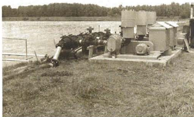
front view of the installed Air Control & Distribution Manifold: Sewer Lagoon Aeration System.
