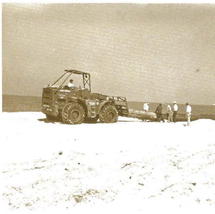
10-Ton Fork Lift Installing Section of Shore Pipe
