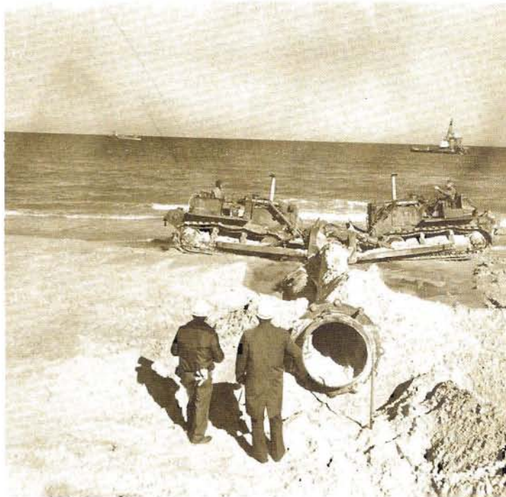
D-7 Bulldozers Removing Shore End of Submerged Pipeline
