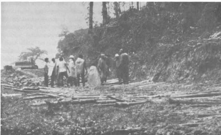
Ecuadorians lay a base course of logs—the palizada on which the finished road will "float".
