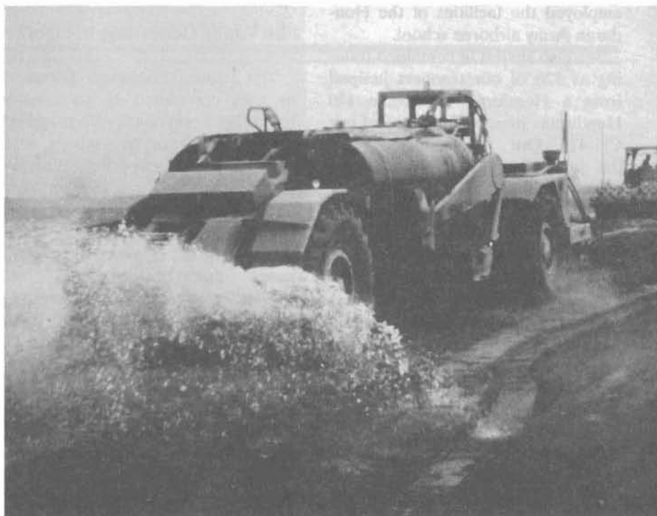
The 27th Engineer Battalion's rapid cement application methods enabled them to cut work time by 75 percent.
