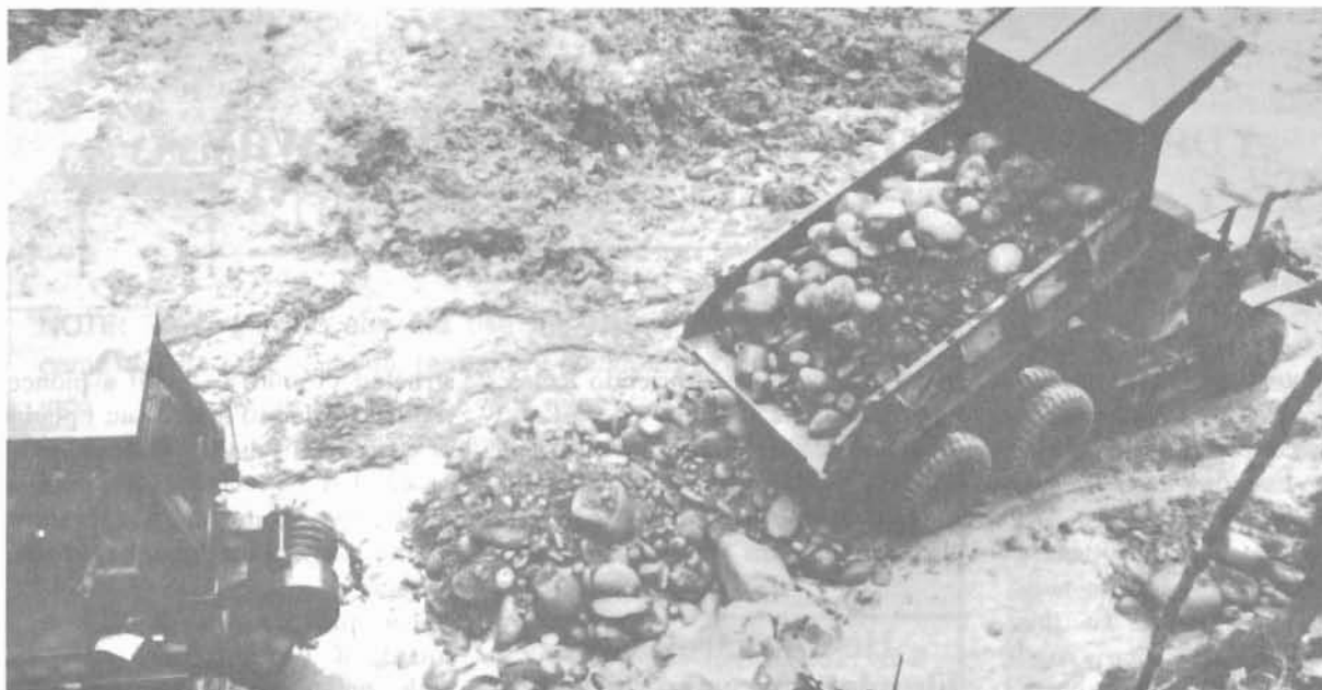
Ecuador's mountain-fed rivers are full of well-worn boulders, excellent material for building roads.
