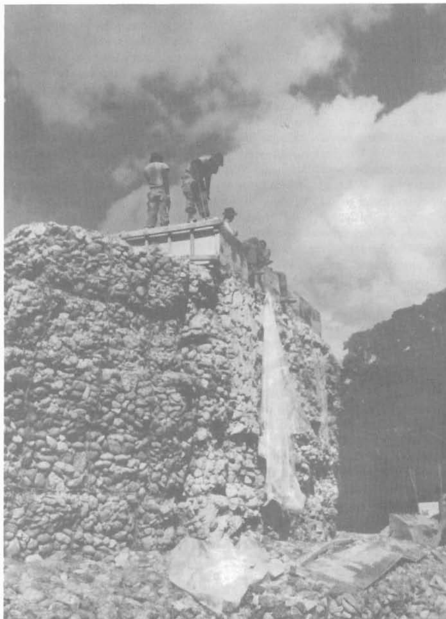
Soldiers loosen the concrete forms that top off a bridge abutment constructed with gabions—rock filled wire baskets.
