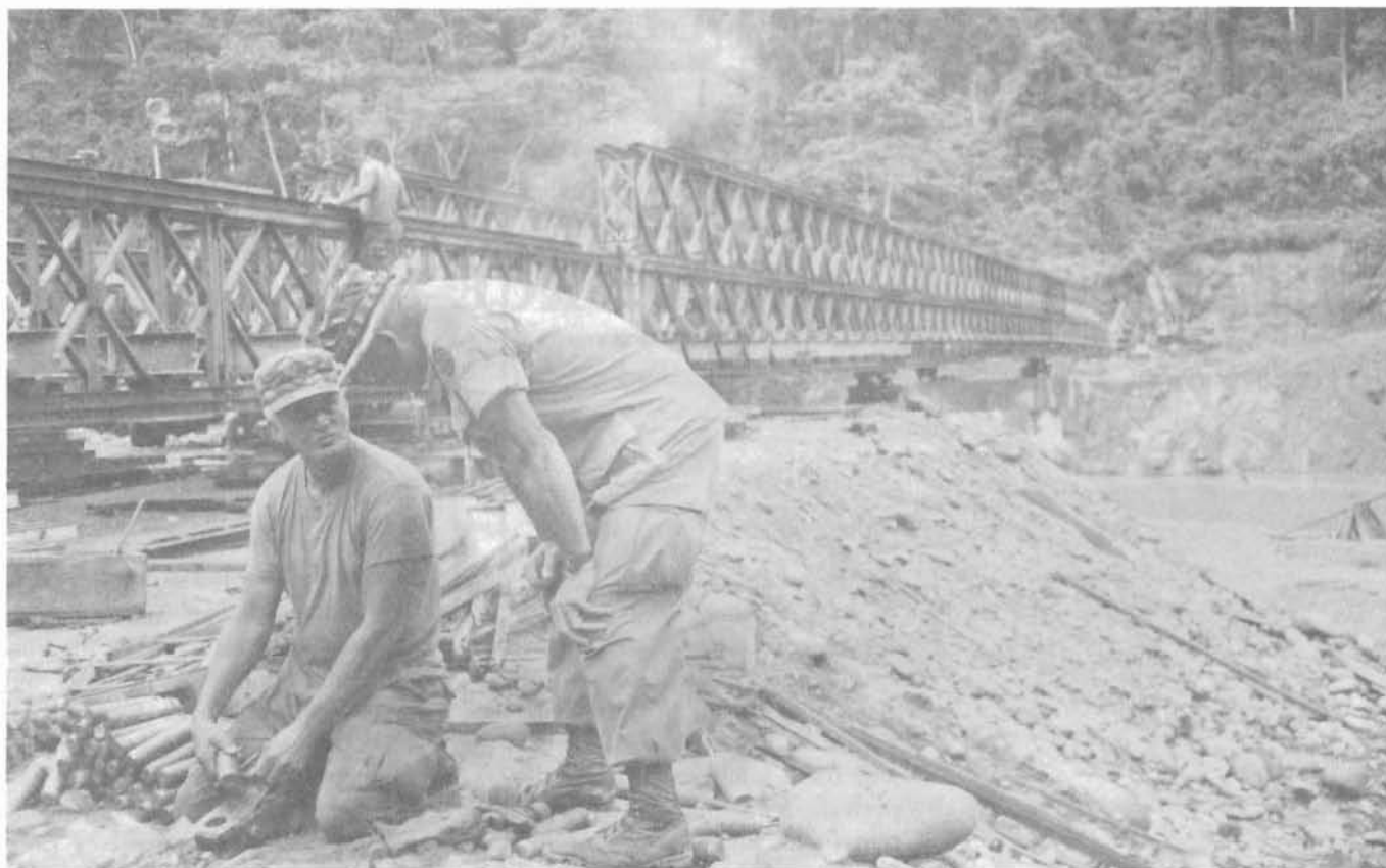
1SG Charles Smitherman and an Alabama National Guardsman consult over chess for the 300-foot ACROW bridge that stretches toward the far bank of the Rio Hollin.
