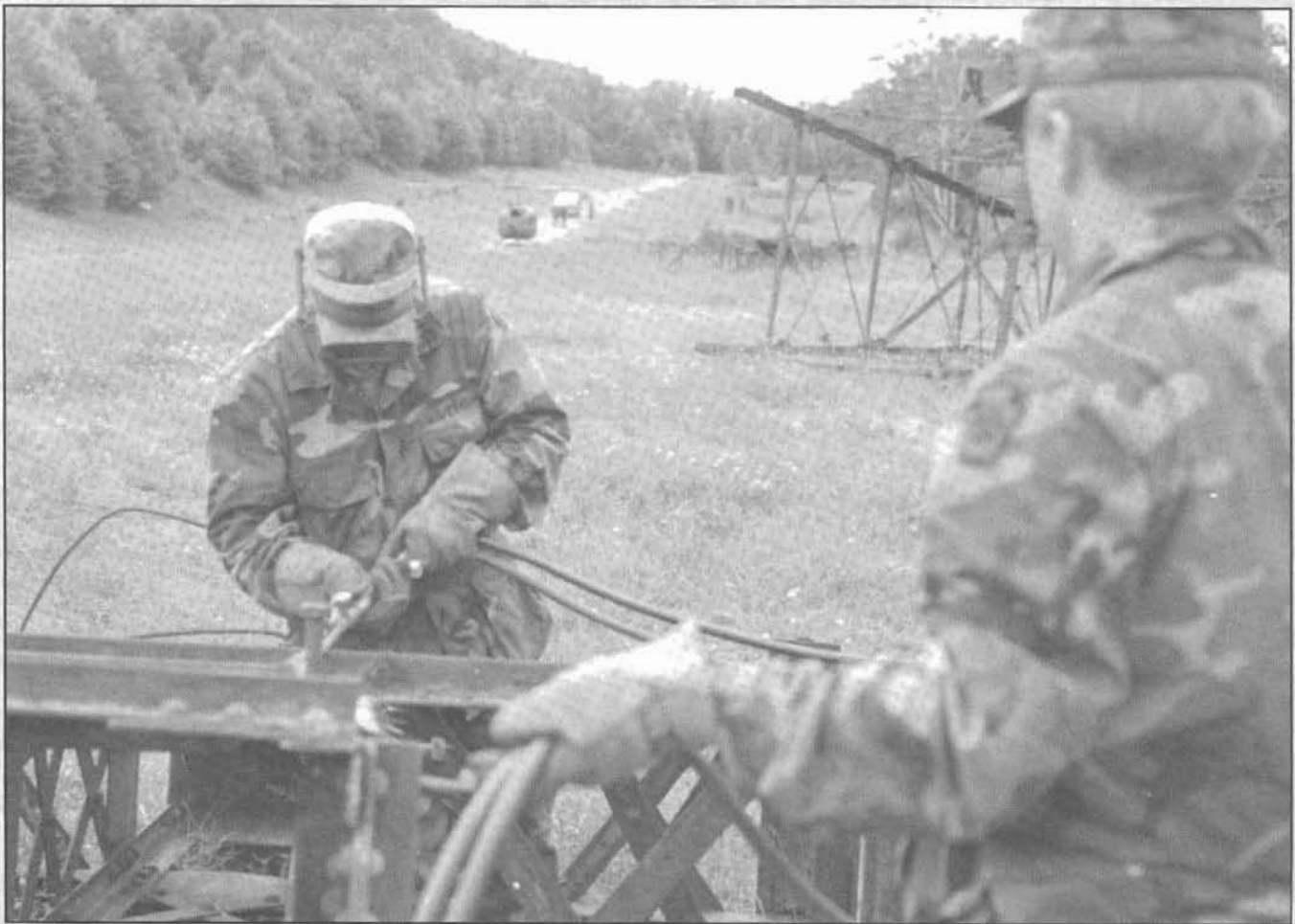
Engineers from the 876th Engineer Battalion, Pennsylvania National Guard, cut steel towers into sections before transporting them to a scrap dealer.
