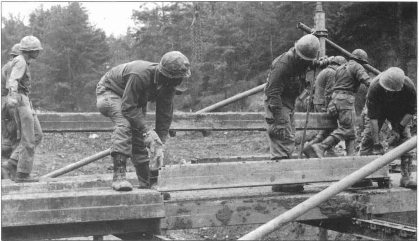
A "team" constructing an M4T6 deck balk bridge with intermediate support. (U.S. Army photo.)
