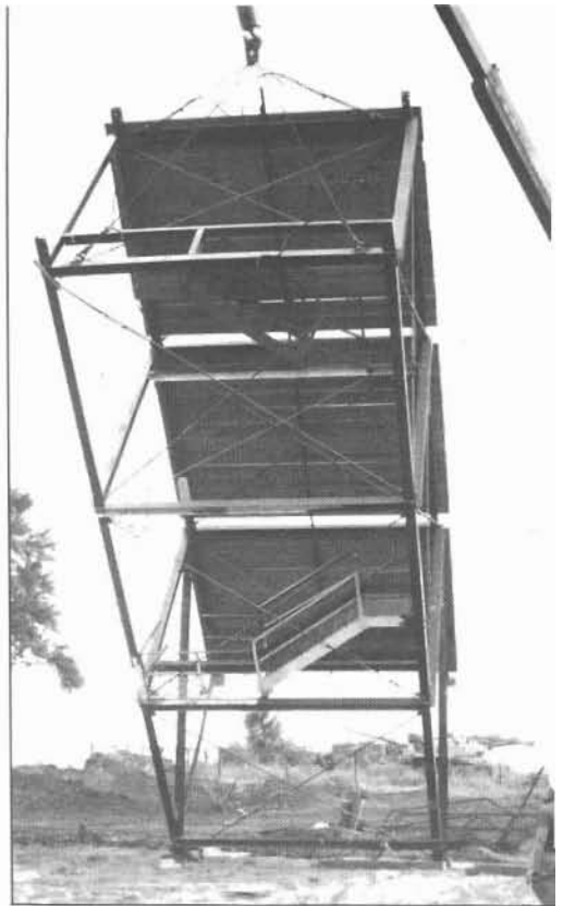
A crane raises a modular tower section onto a new foundation.
