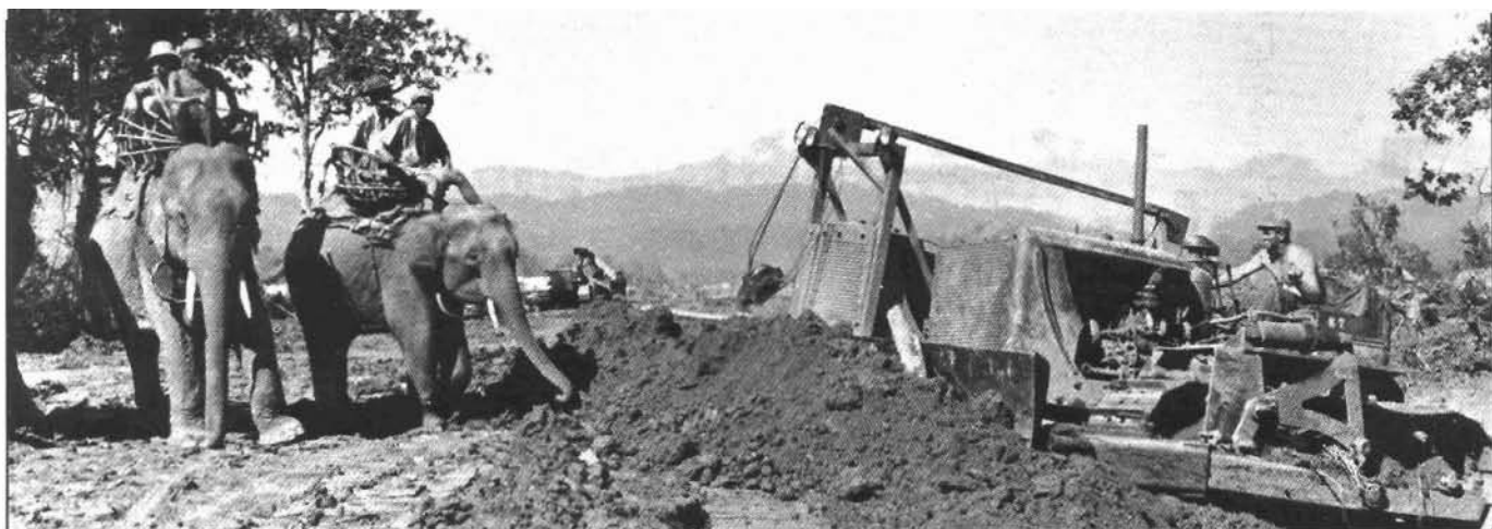
A survey party on elephants passes a bulldozer working on the Ledo Road in northern Burma. The 500-mile road was constructed by U.S. Army engineers during World War II to connect northeastern India with the Burma Road leading into southwestern China (U.S. Army photo).
