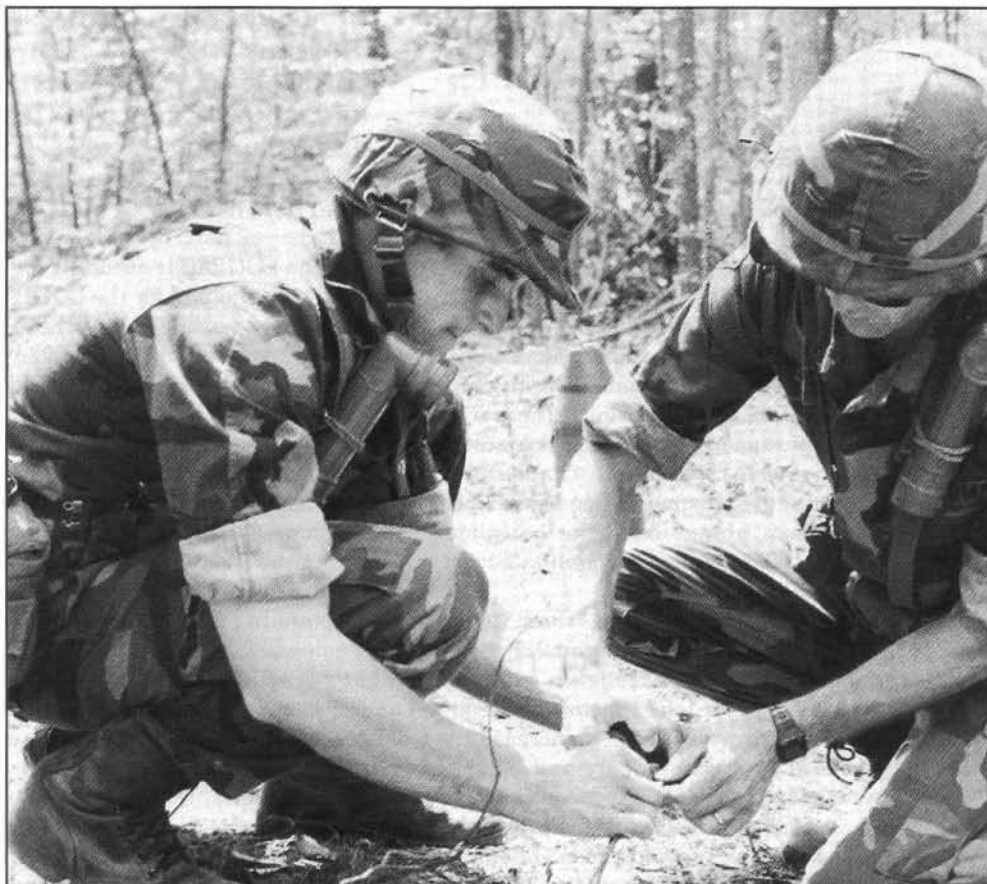
Priming a shaped charge, 2LT Jay P. Still and 2LT Michael L. Rogers prepare to detonate explosives to create a hasty road crater. Demolitions is one of the many challenging tasks for EOBC students during an FTX at Fort A.P. Hill, VA (photo by 1LT L. J. Leto).
