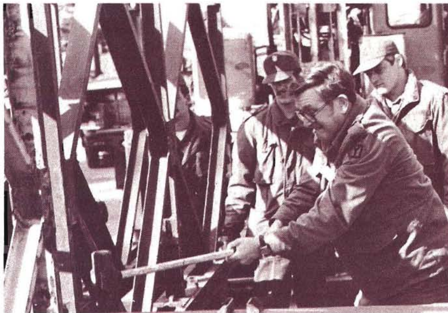
Platoon Sergeant Richard McBain drives home a connector on a Bailey Bridge which his Massachusetts National Guard Unit—Company B, 101st Engineer Battalion, 26th (Yankee) Infantry Division—constructed recently as a temporary replacement for the condemned Pearl Street Bridge in Lowell, MA. More than 75 citizen-soldiers of Company B and Headquarters Company turned out for the weekend training and community assistance project. (Photo by SP5 Thomas J. Spisak)
