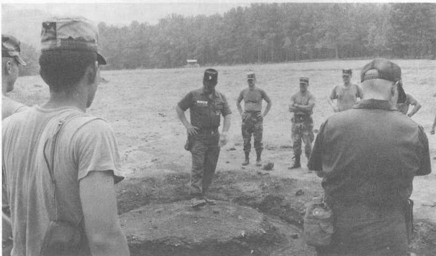
Mr. Roger Boyd examines the preliminary groundwork prepared for the simulator device.
