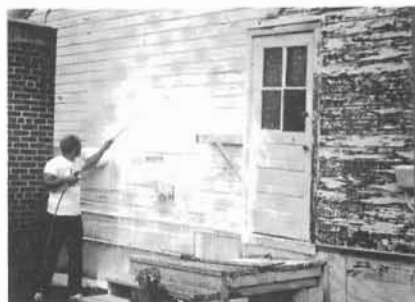
Loose paint is removed from a wood structure during a CERL test.
