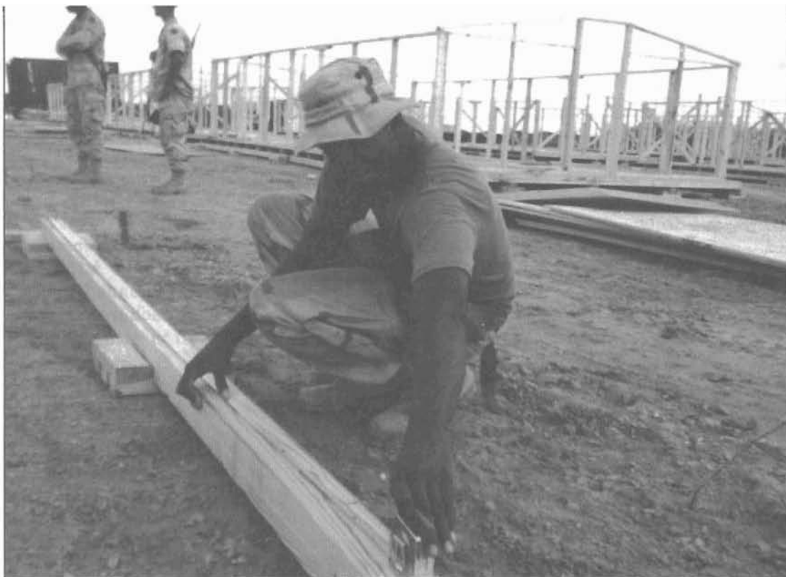
PV2 Mebane of 1st platoon, B Company, marks floor joist positions on a strongback tent beam.
