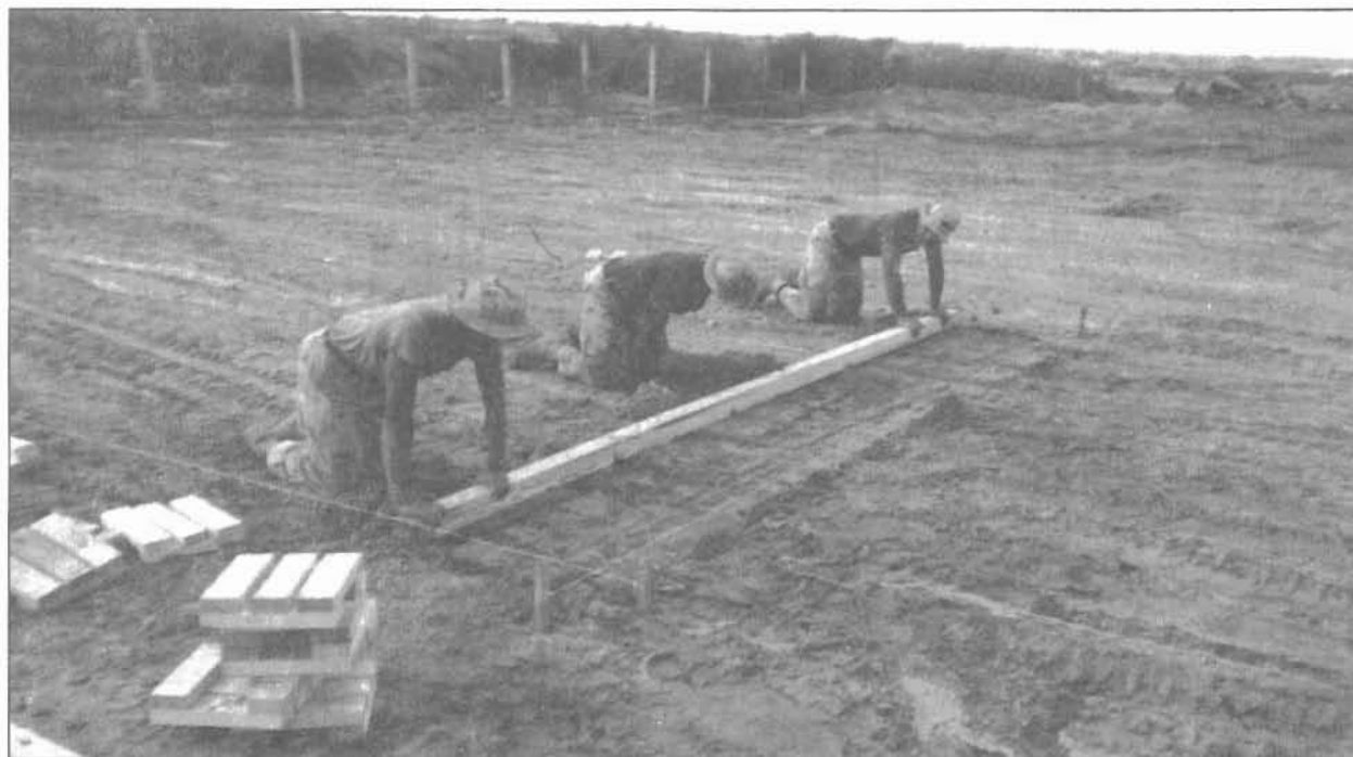
SPC Martin, SPC Fullwood and SPC Massey (left to right) of 1st platoon, B Company, level the ground prior to placing strongback footings.
