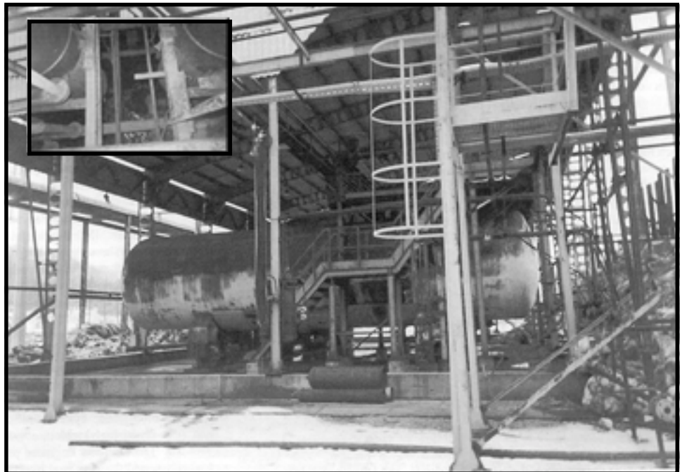
The Sudaso Chemical Plant near Tuzla; inset shows a spill of liquid mercury inside the plant.
