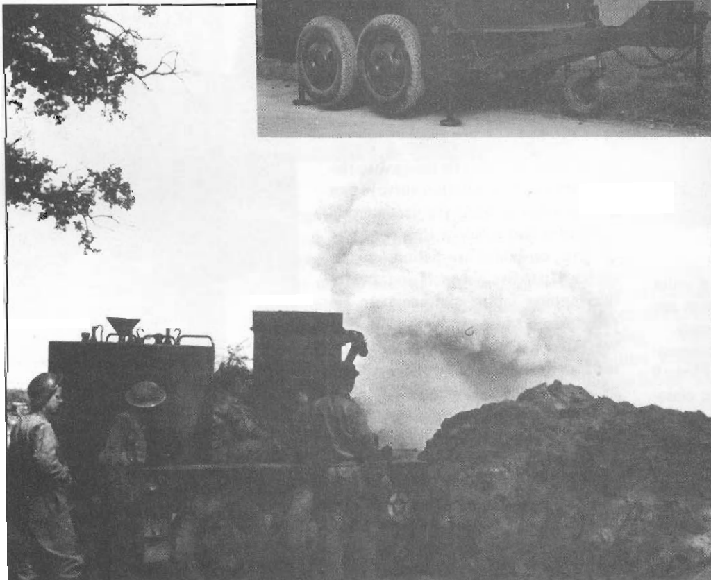
The M1 smoke generator (inset and below) weighed 3,000 pounds empty and 5,400 pounds filled.
