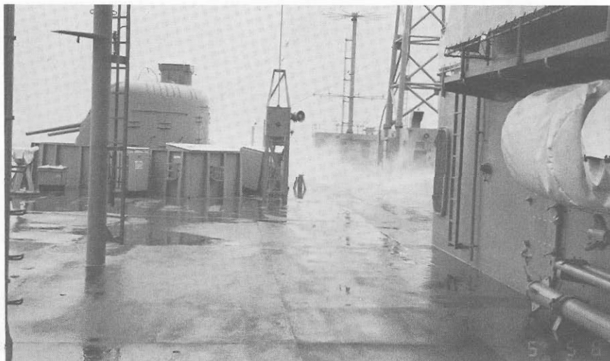
Ship's water washdown system flushes chemicals from deck.
