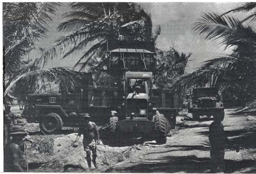
CLEAN-UP OPERATIONS ON MEDREN
