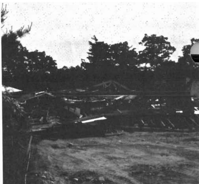
Engineers from the 18th raze some old buildings to make the post look beautiful.
