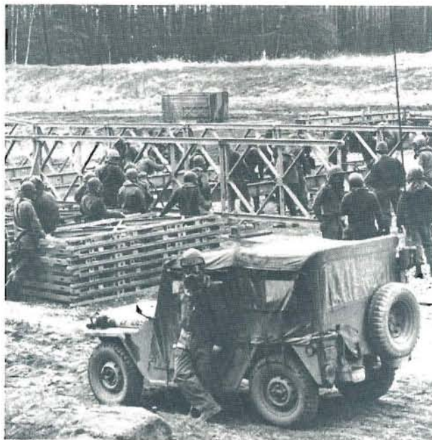
During the administrative phase, engineer troops integrated CBR with Bailey Bridge construction.
