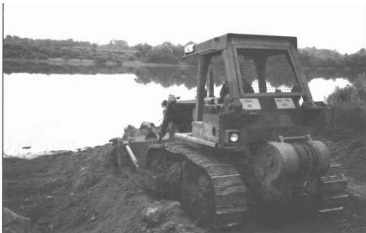
A bulldozer from the 535th CSE prepares ramps at the Sava River to support the division's redeployment to Germany.
